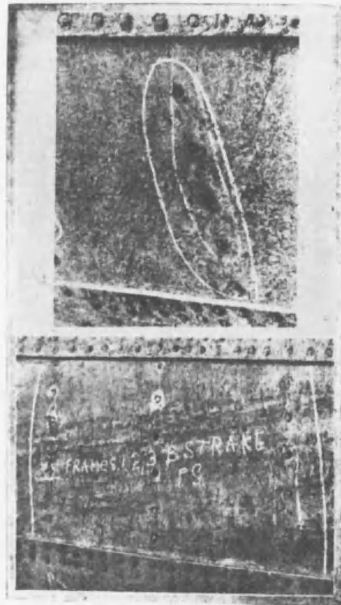
Typical cases of corroded steel rivet points.
