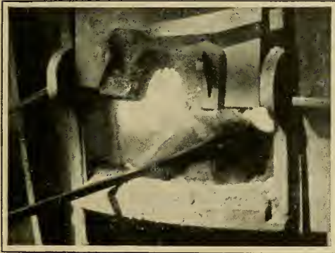
TURNING THE PIGS TO INSURE EVEN MELTING
