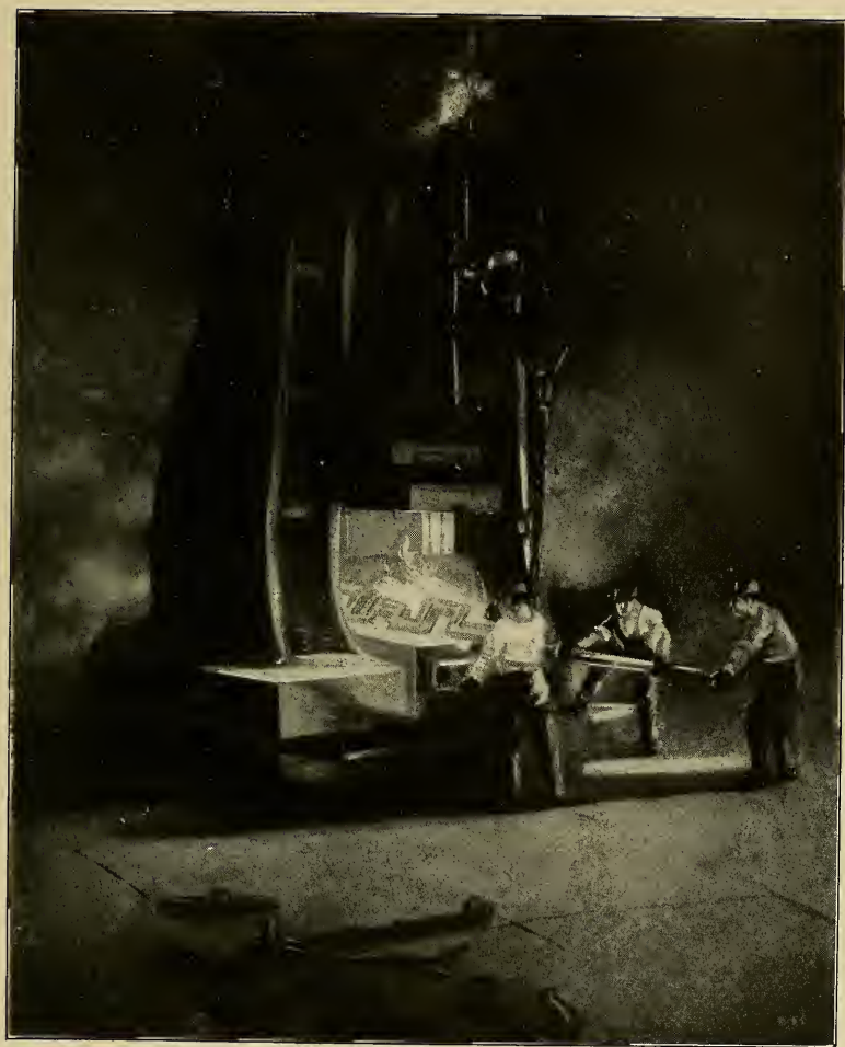
MODERN FORGING OF AN AUTOMOBILE CRANK SHAFT
