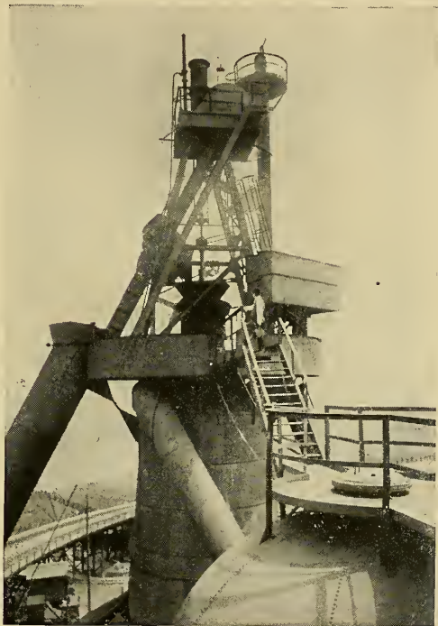
SKIP HOIST AT WORK. SKIP DUMPING INTO HOPPER
