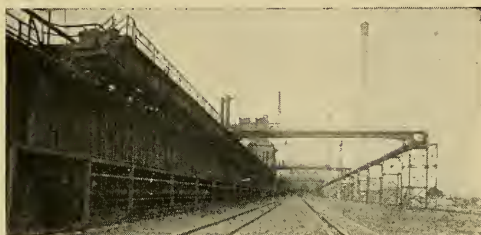
BATTERY OF BY-PRODUCT COKE OVENS, SHOWING GAS-COLLECTING MAIN
