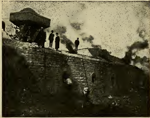
CHARGING COAL INTO THE OVENS
