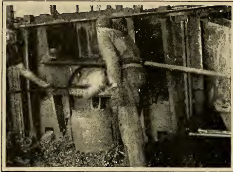
PUDDLING THE MELTED CHARGE
