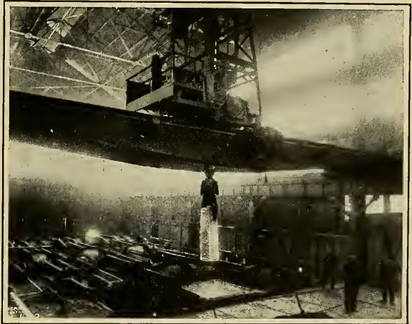
INGOT COMING OUT OF THE "SOAKING PIT"
