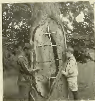
One Davy method of reinforcing cement
