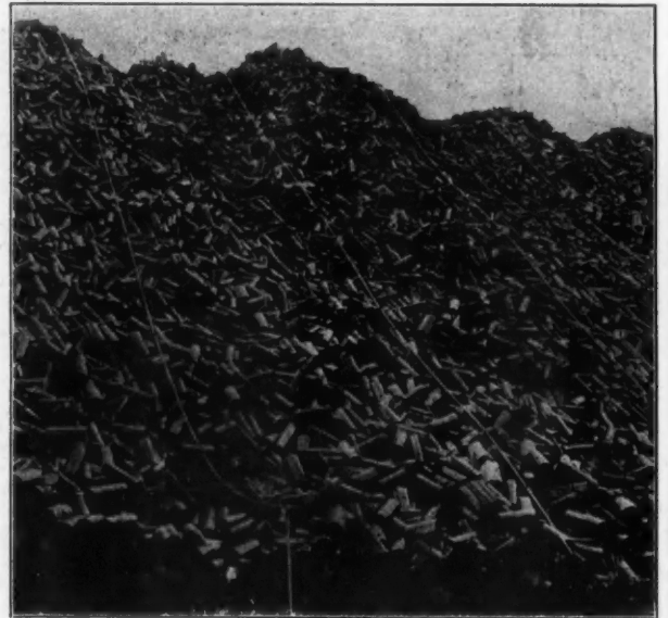
FIGURE 14. LOG PILE CONTINUOUSLY WET BY SPRAY NOZZLES MADE OF BRASS \frac{1}{2} -IN. PIPE CAPS WITH THREE \frac{1}{32} -IN. HOLES SPACED 25 x 30 FEET.
