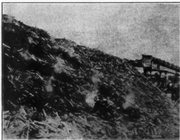
FIGURE 15. SPRAY NOZZLES USING 2 QUARTS OF WATER PER MINUTE EACH SPACED 30 FEET EACH WAY. THE SURFACE IS NOT QUITE COVERED DUE TO THE UNEQUAL DISTRIBUTION FROM INSUFFICIENT ELEVATION.
