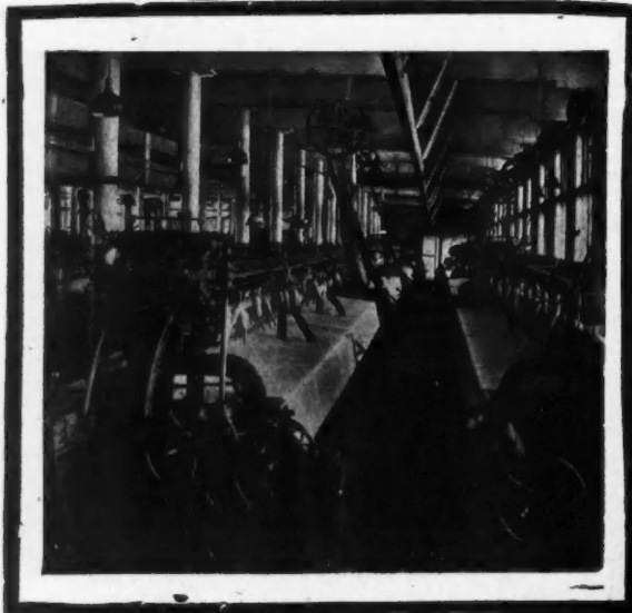
Joining by hand the two ends of woven fabric into felts.
