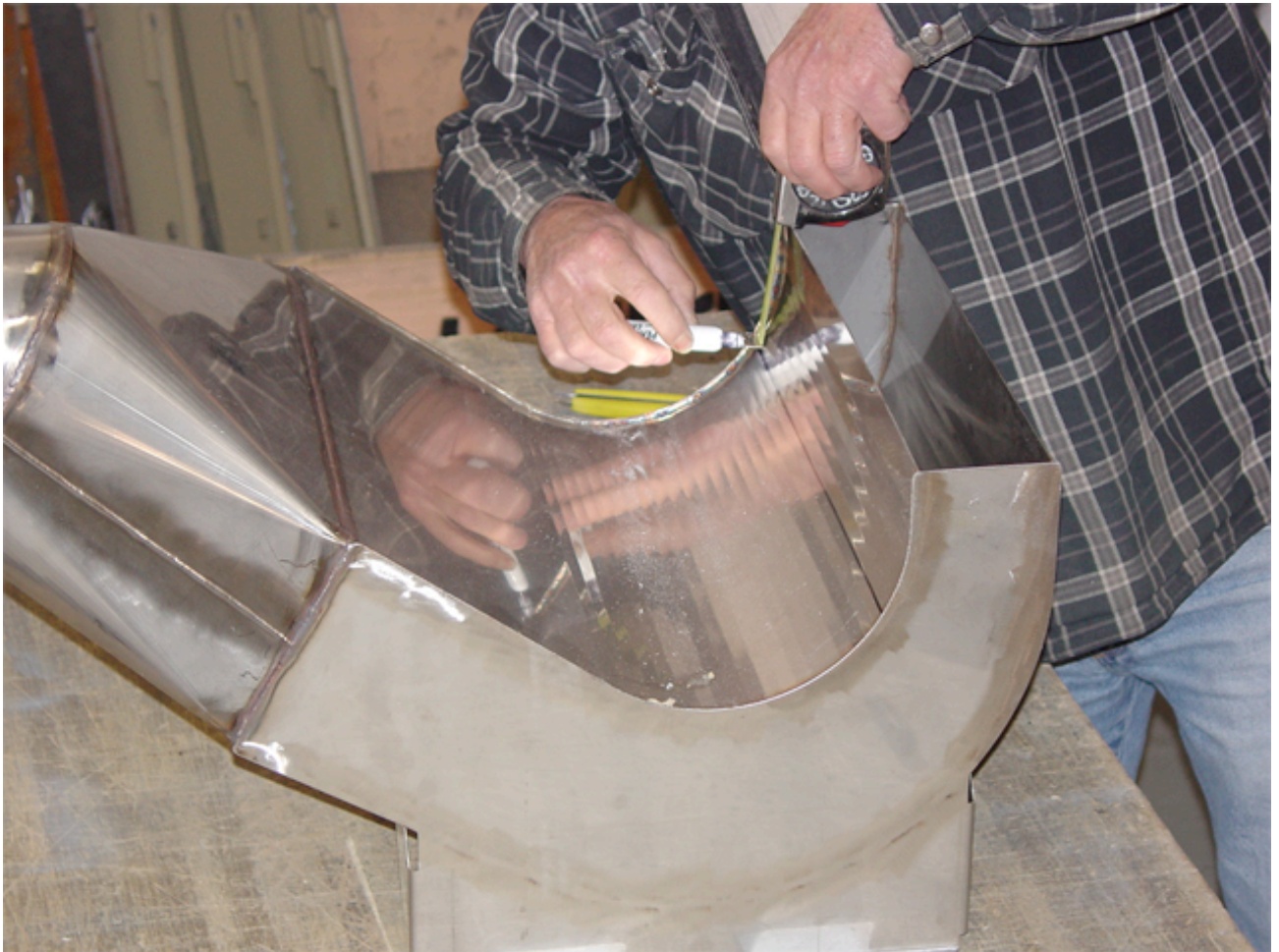
Figure 8. Measuring the Plenum.
