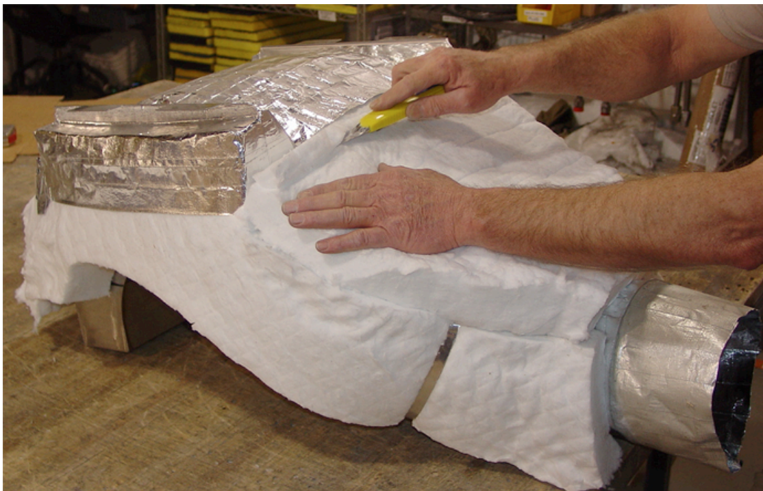
Figure 21. Trimming Insulation from Plenum (Sheet 2 of 2).
