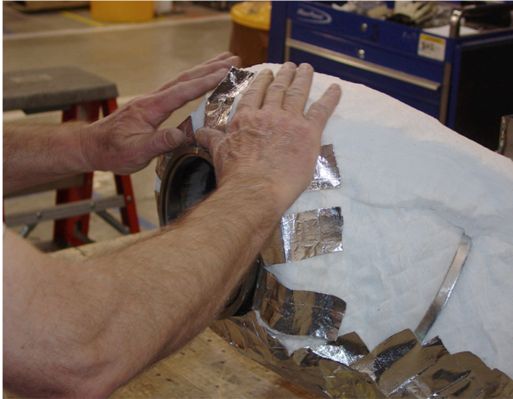
Figure 27. Attaching Top Piece of Insulation to the Rest of the Insulation (Sheet 1 of 2).
