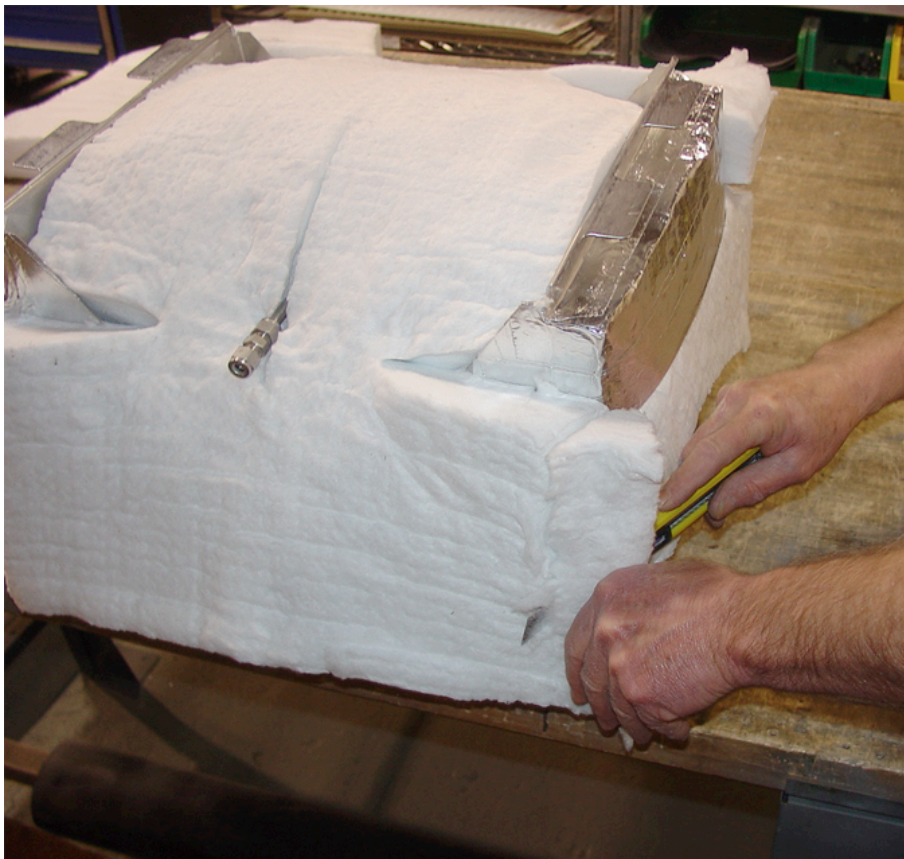
Figure 18. Trimming Insulation on the Plenum (Sheet 1 of 2).
