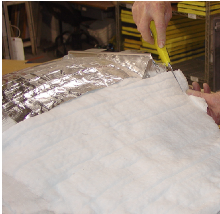
Figure 21. Trimming Insulation from Plenum (Sheet 1 of 2).
