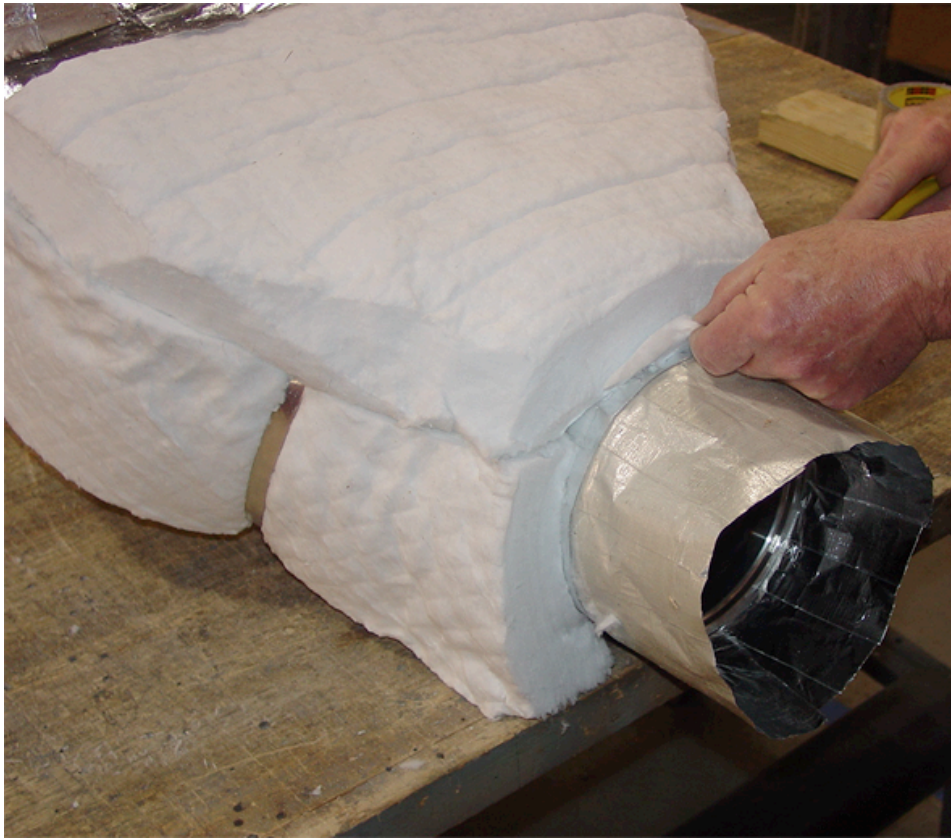
Figure 22. Trimming Insulation Around the Inlet (Sheet 2 of 2).
