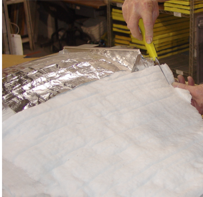
Figure 22. Trimming Insulation Around the Inlet (Sheet 1 of 2).
