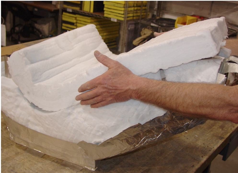
Figure 25. Snugging Insulation into the Bend (Sheet 1 of 2).
