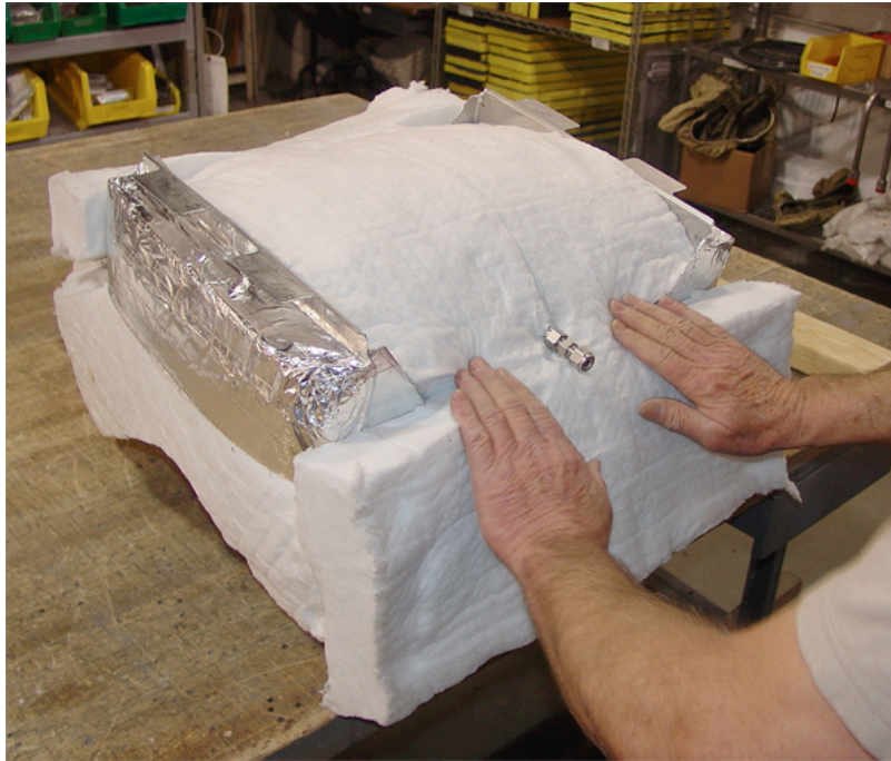
Figure 17. Placing Insulation on the Bottom of the Plenum Showing the Extension Tube.
