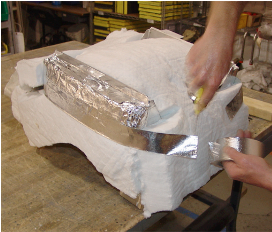
Figure 18. Trimming Insulation on the Plenum (Sheet 2 of 2).
