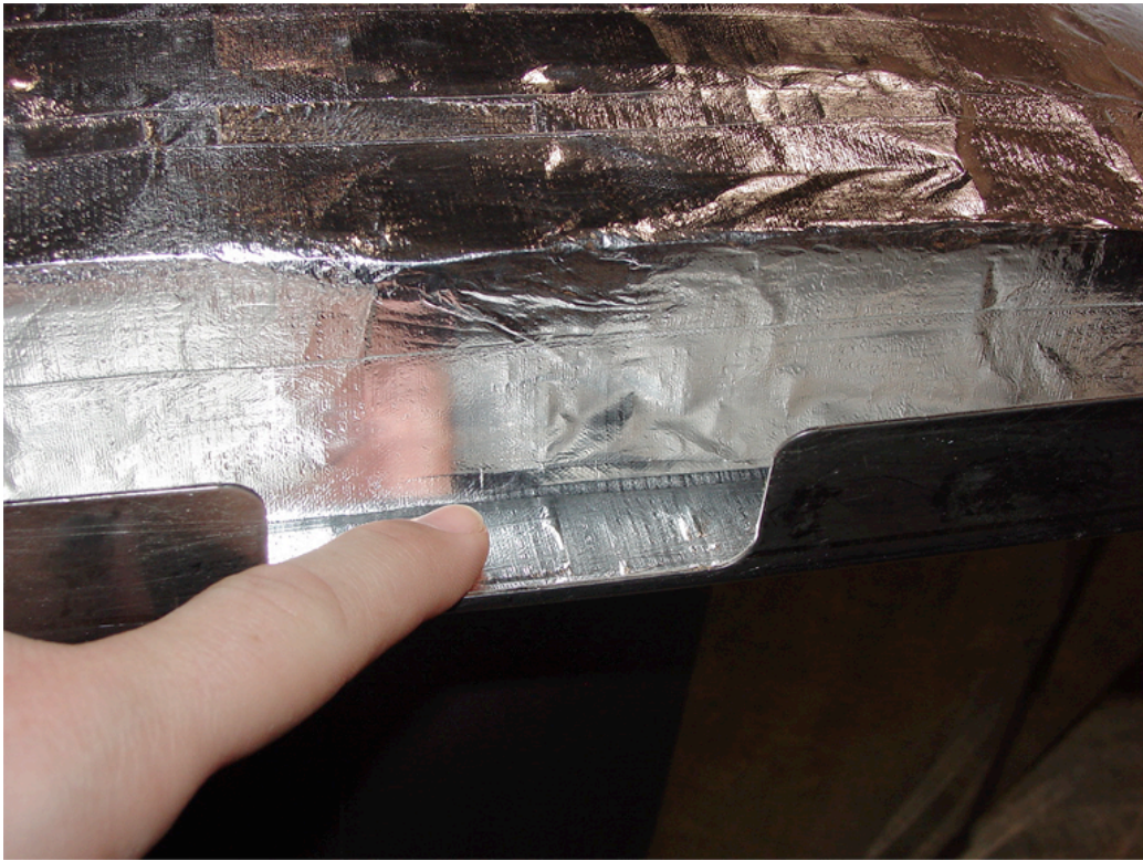
Figure 14. Taping of the Plenum (Bottom).
