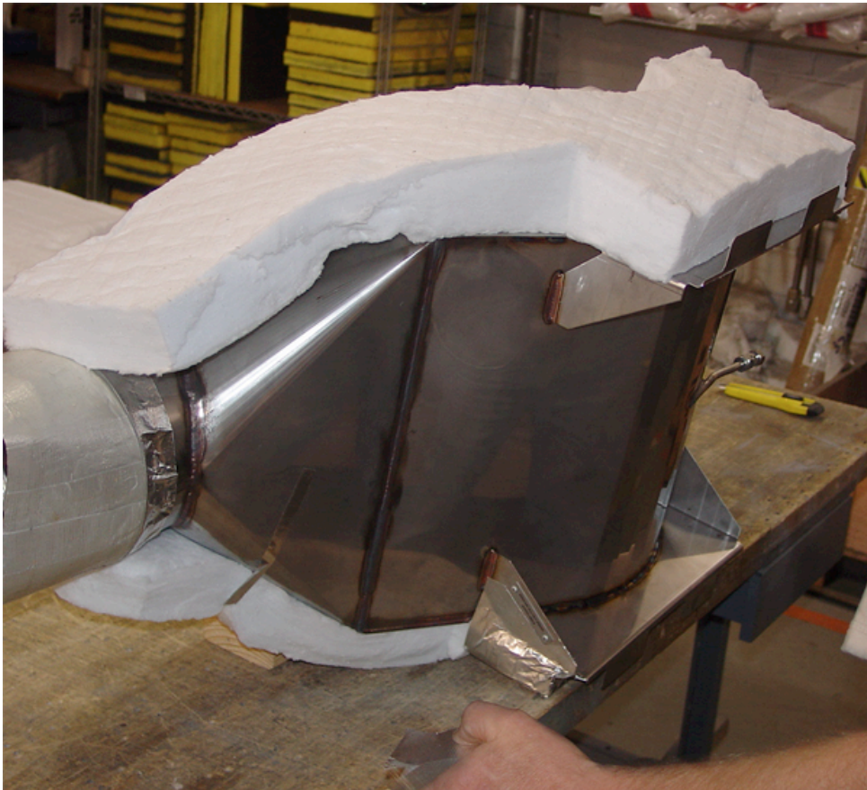
Figure 15. Preparing Insulation for Taping (Sheet 1 of 2).
