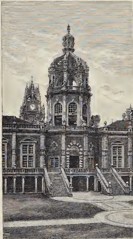
No. 5.—Water Tower between Hall and Kitchen. Engraved by J. J. Cocking.
