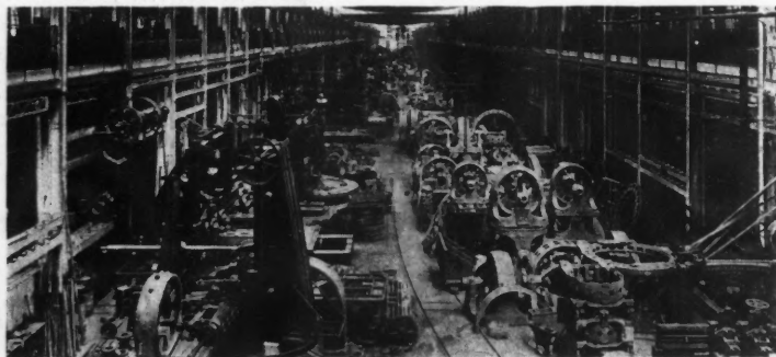
The manufacturing plants of Pennsylvania are the safest and most modern in the world. This is an electrical shop in the Pittsburgh district
