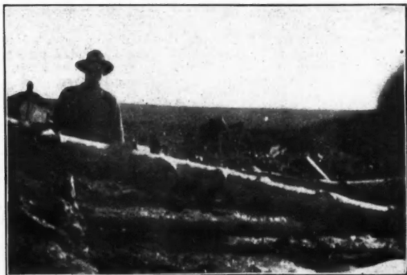
UPPER END, WITH CREW AT WORK.
