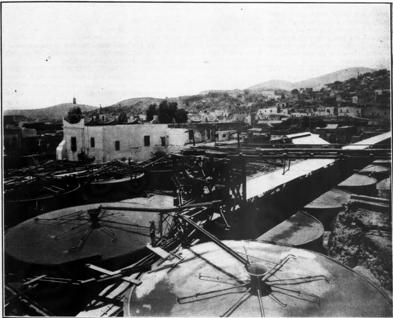
FIG. 4. ARRANGEMENT OF TANKS, FLORES CYANIDE PLANT, GUANAJUATO
