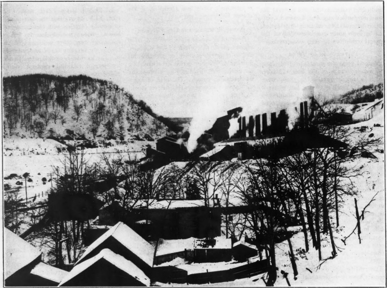
SURFACE PLANT, ST. CLAIR COLLIERY, ST. CLAIR, PENN.
