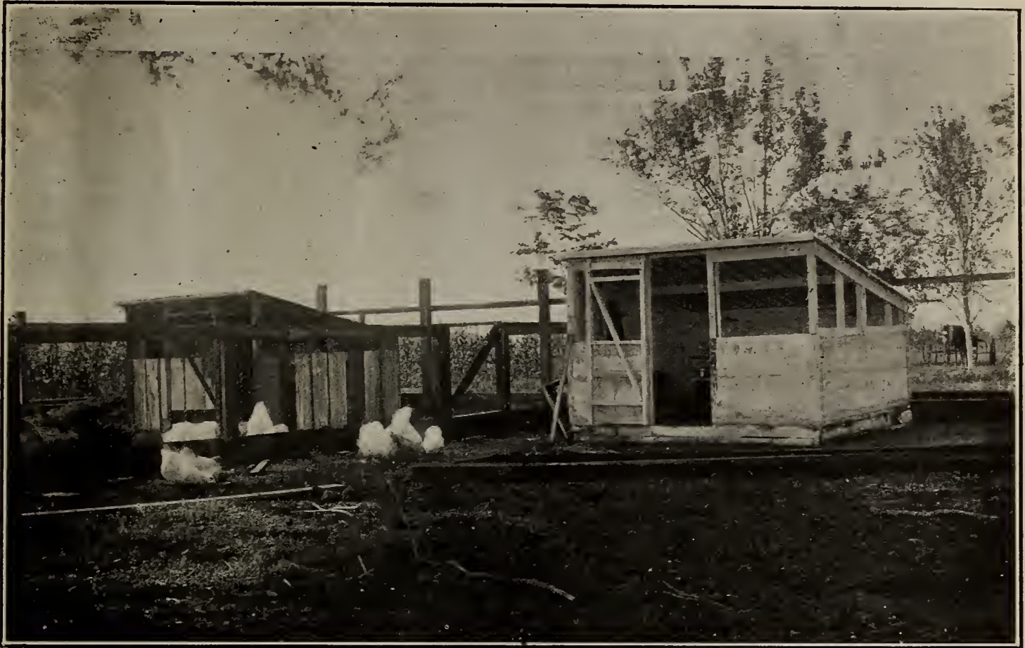
Showing Construction of Hen Houses, Bellevue Poultry Farm, Jeanerette, La.
