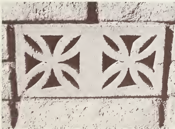
Figure 7. Decorative concrete vent block.
