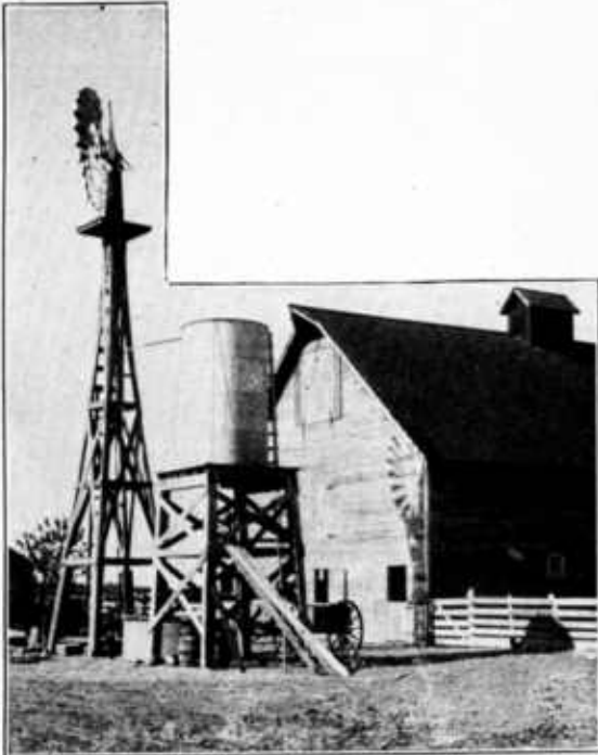
FIG. 42.—Galvanized-iron tank on timber trestle, Herington, Kans. Tank is not used in winter and is unsightly.
