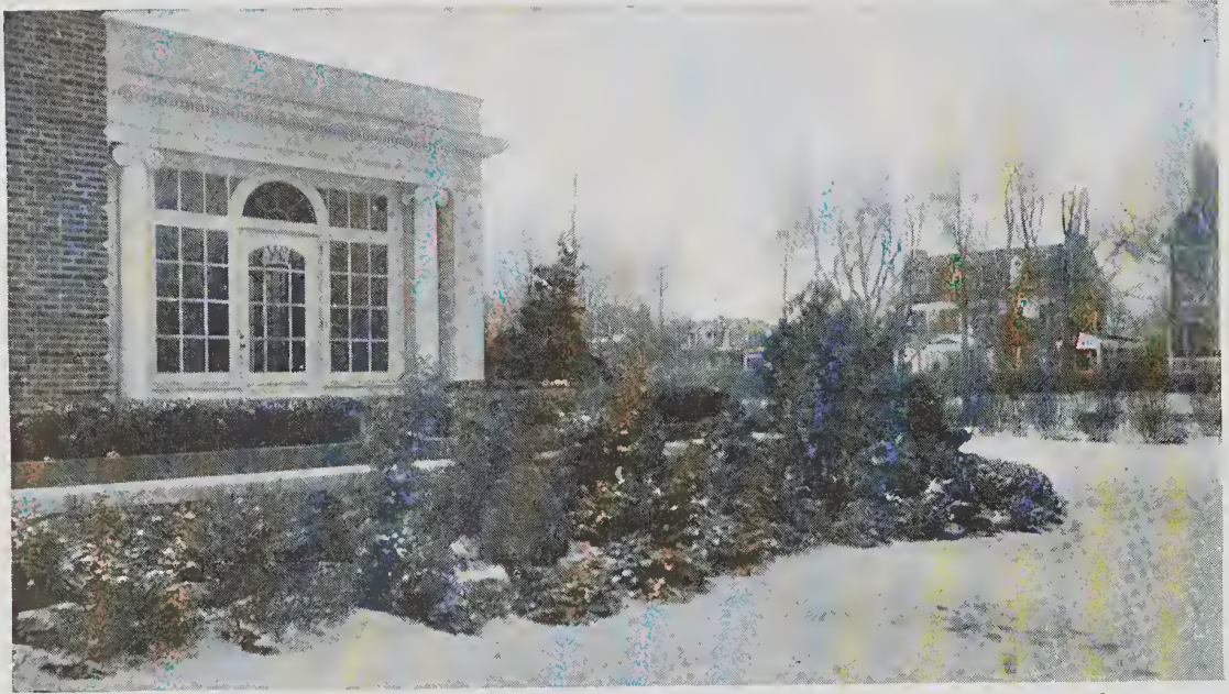
The informal planting of Evergreens successfully softens the base-line of the house and terrace
