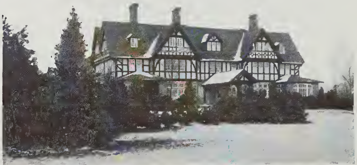
Planting of Evergreens completely screening the service end of the house
