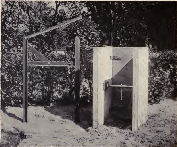
MARK V SHUTTERING.
