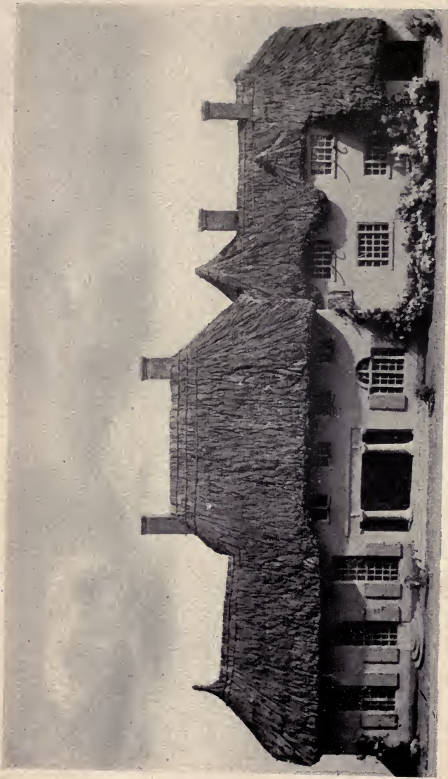
MODEL OF A PISÉ DE TERRE HOUSE TO BE BUILT IN THREE SUCCESSIVE STAGES. The right wing is planned to be built first as a complete small cottage, eventually becoming service and servants' quarters.
