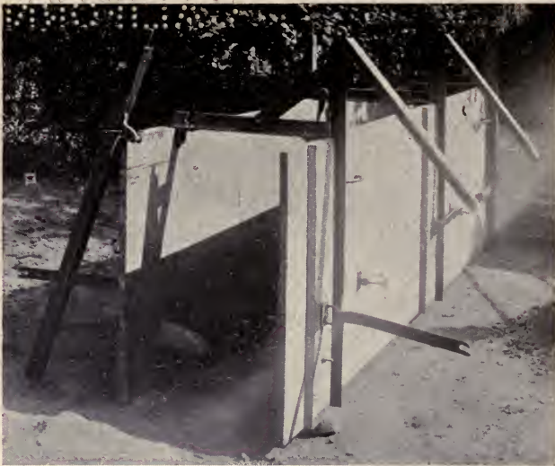
MARK V SHUTTERING.
