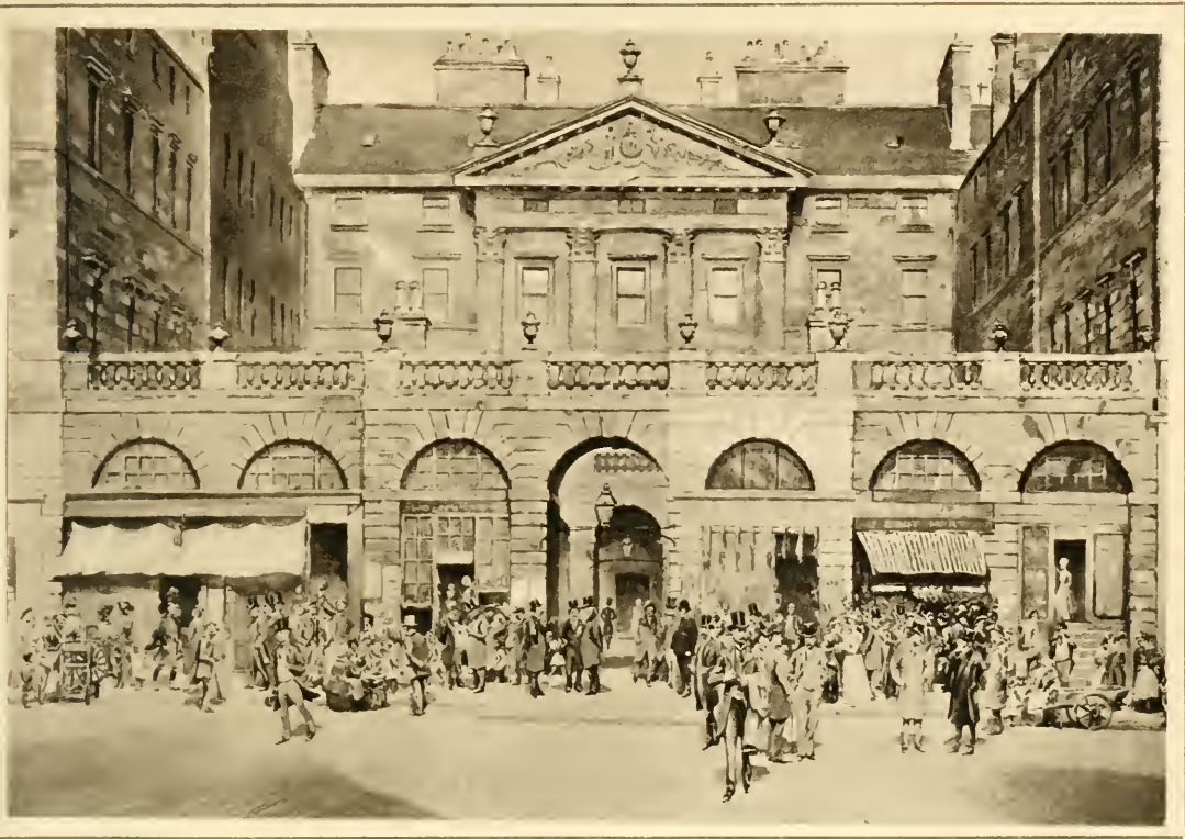
FAÇADE OF ROYAL EXCHANGE
