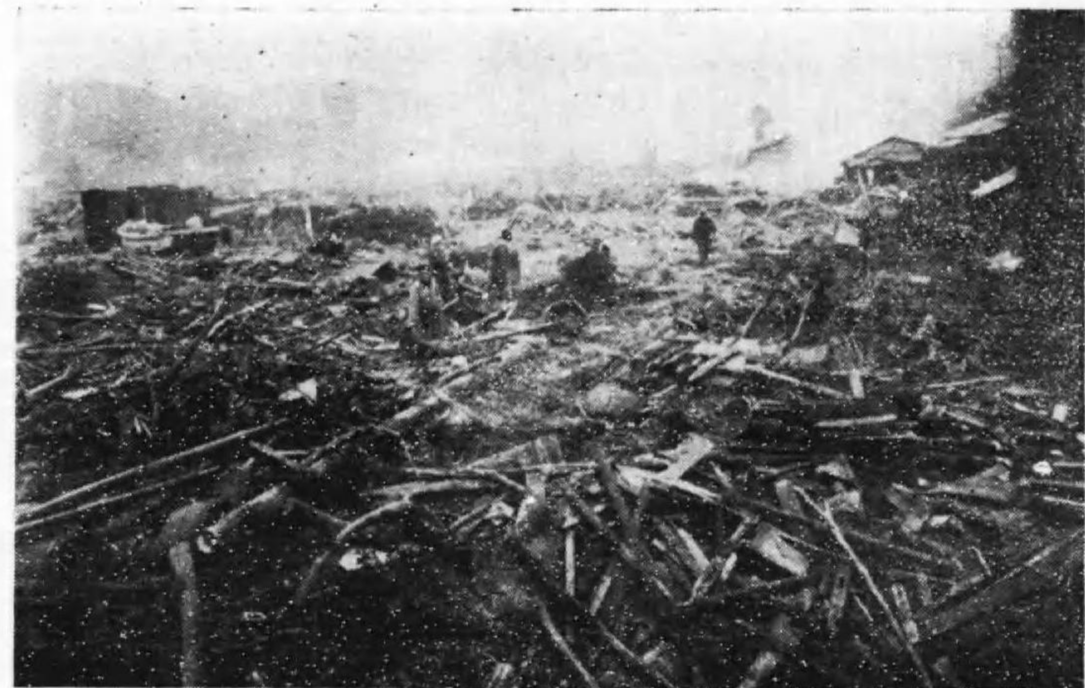
(大槌町被害状況)
