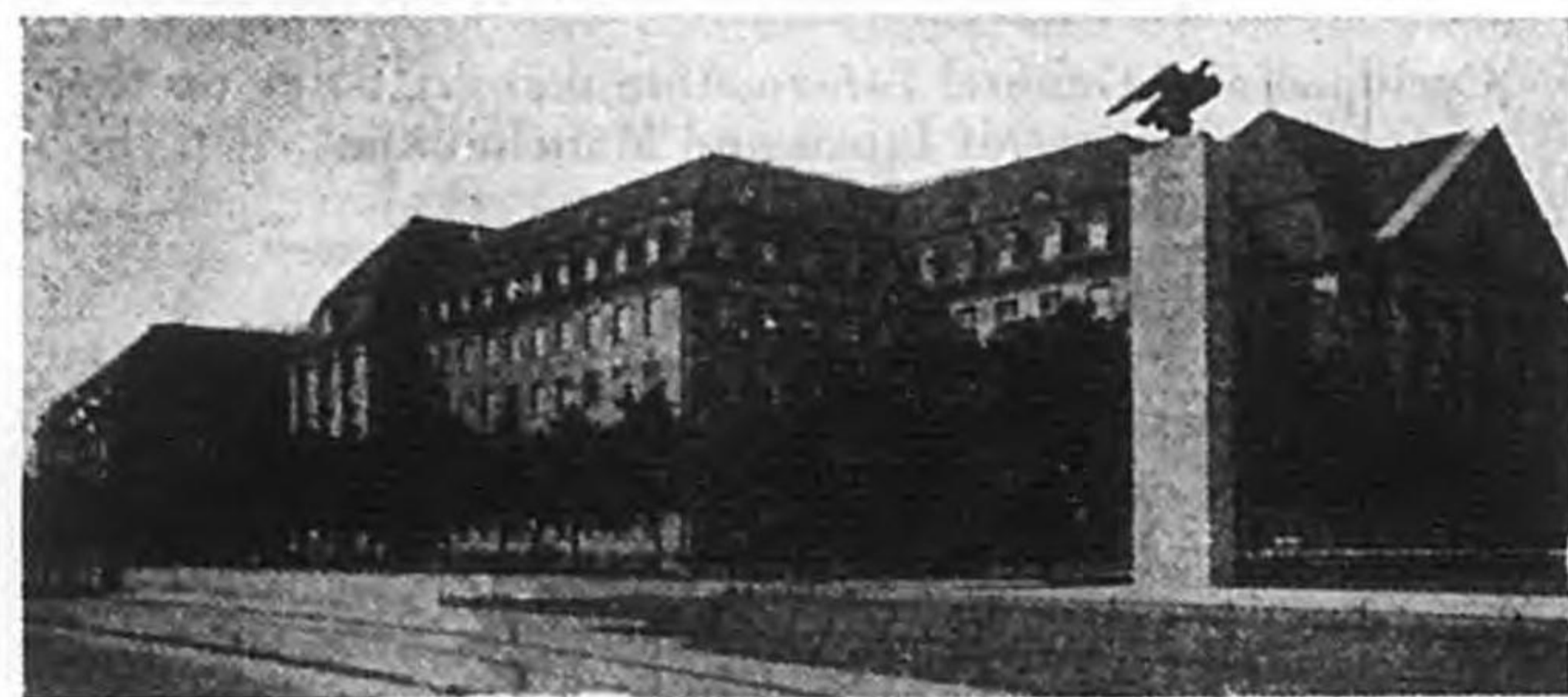
The Head Office-building at Berlin-Siemensstadt
