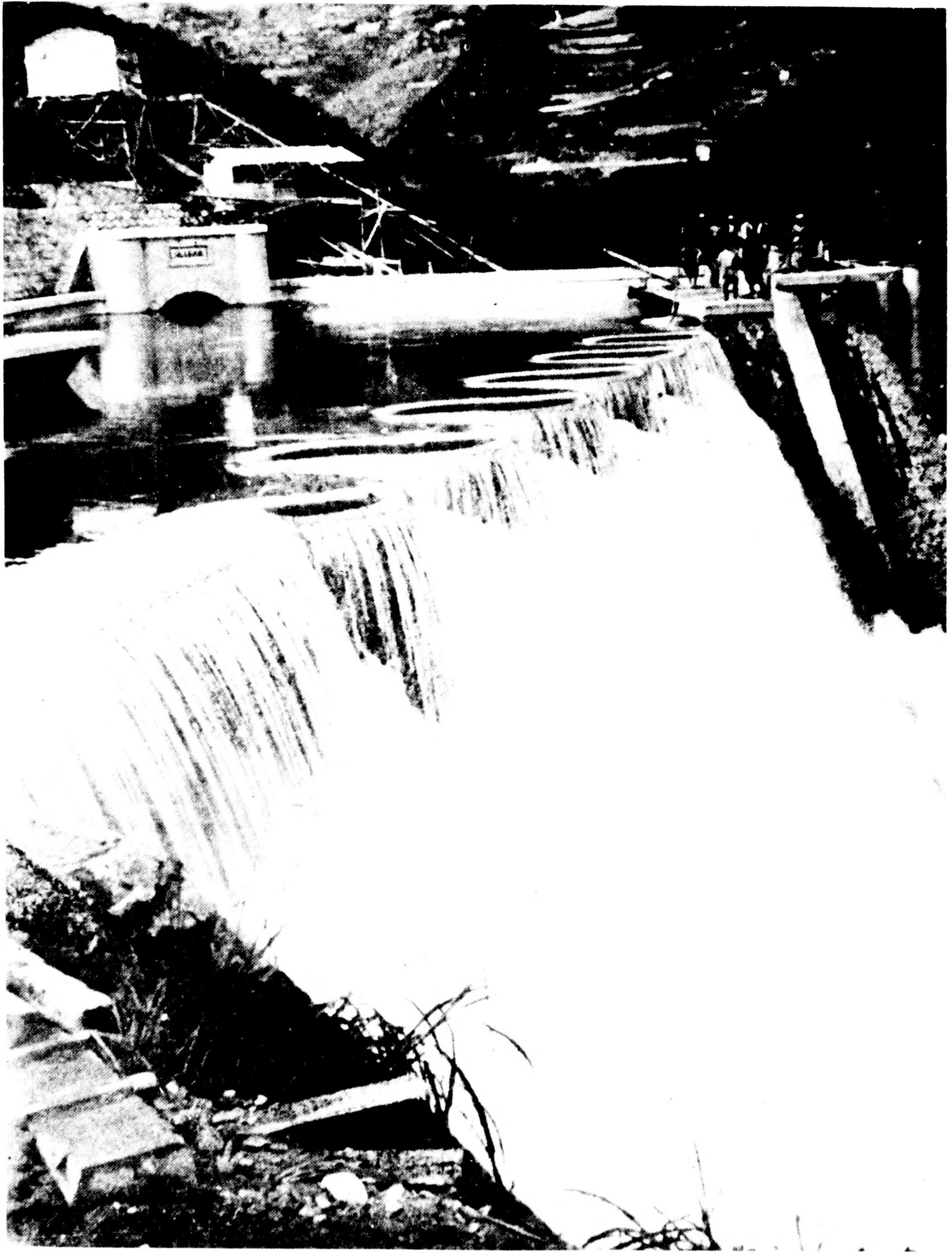
Photograph No. IV-63 Omogo No. 3 Hydro Plant forebay in 1938
