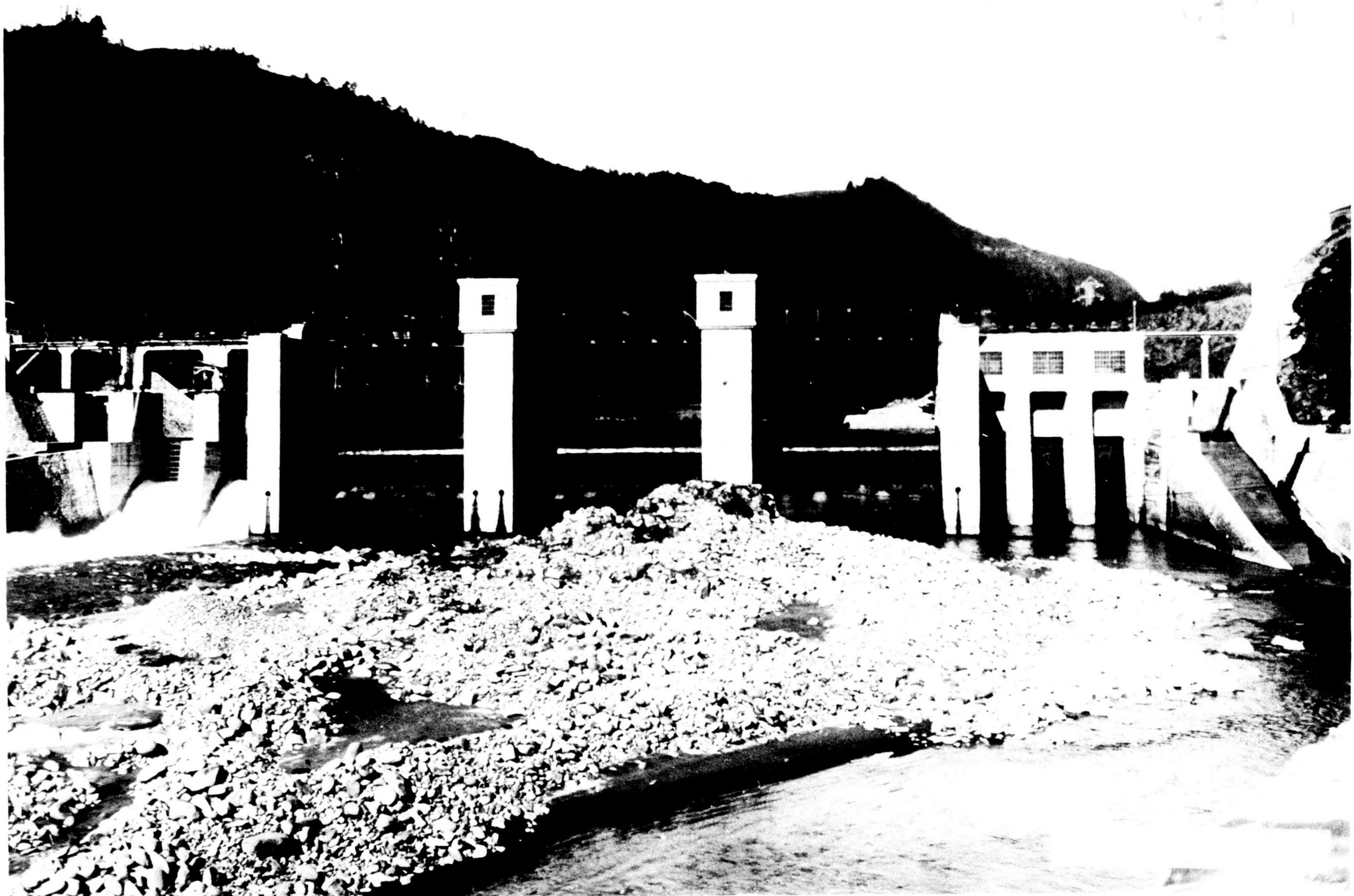
Photograph No. IV-92 Saku Hydro Plant dam
