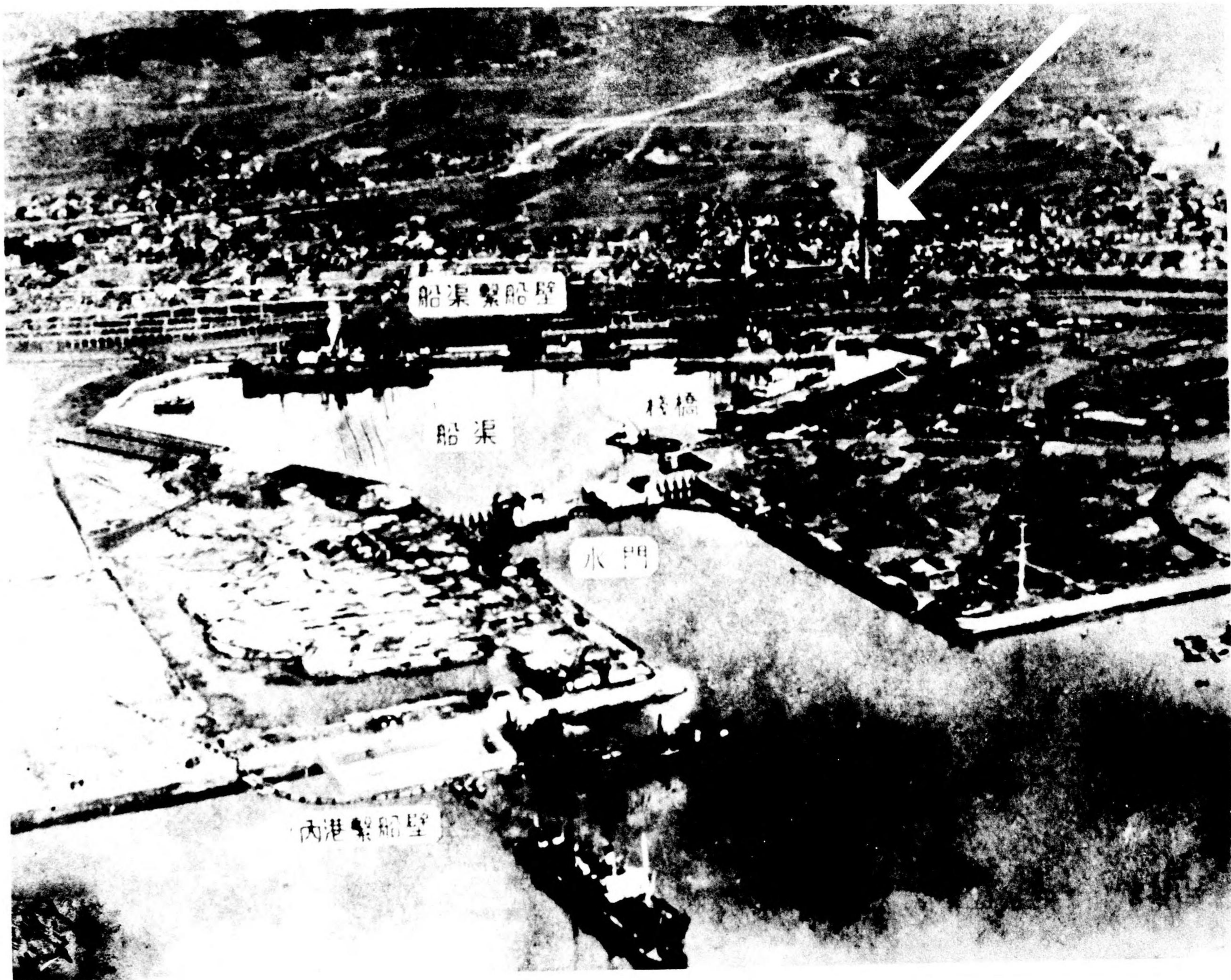
Photograph No. IV-76 Oura Steam Plant (arrow)
