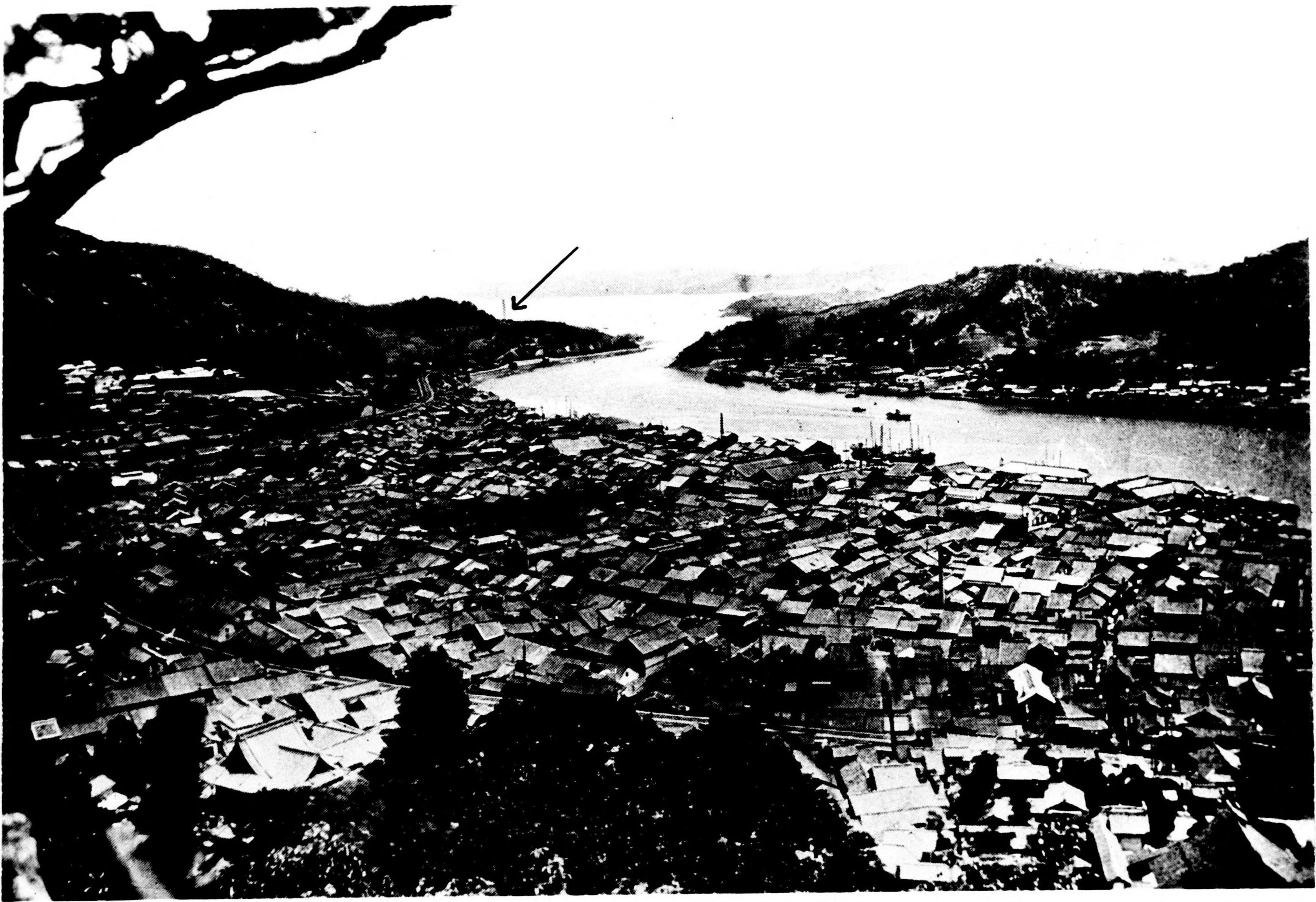
Photograph No. IV-67b Onomichi Steam Plant (arrow) OSS R 112585
