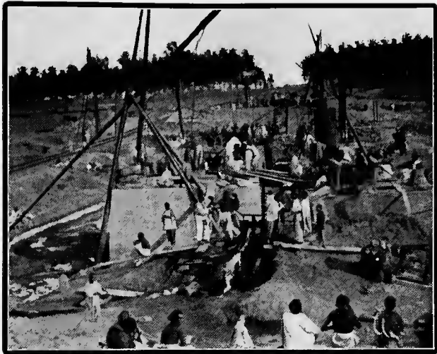
GERMANS BUILDING RAILWAY BRIDGE IN SHANTUNG
