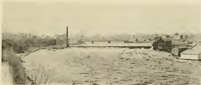
THE WATER WORKS AND DAM
