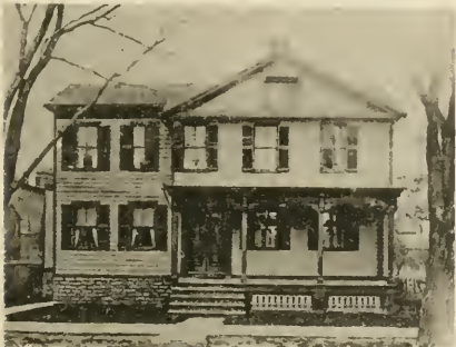
RESIDENCE OF J. Y. CHAPIN
