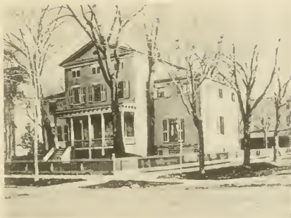
RESIDENCE OF N. P. WOOLEY
