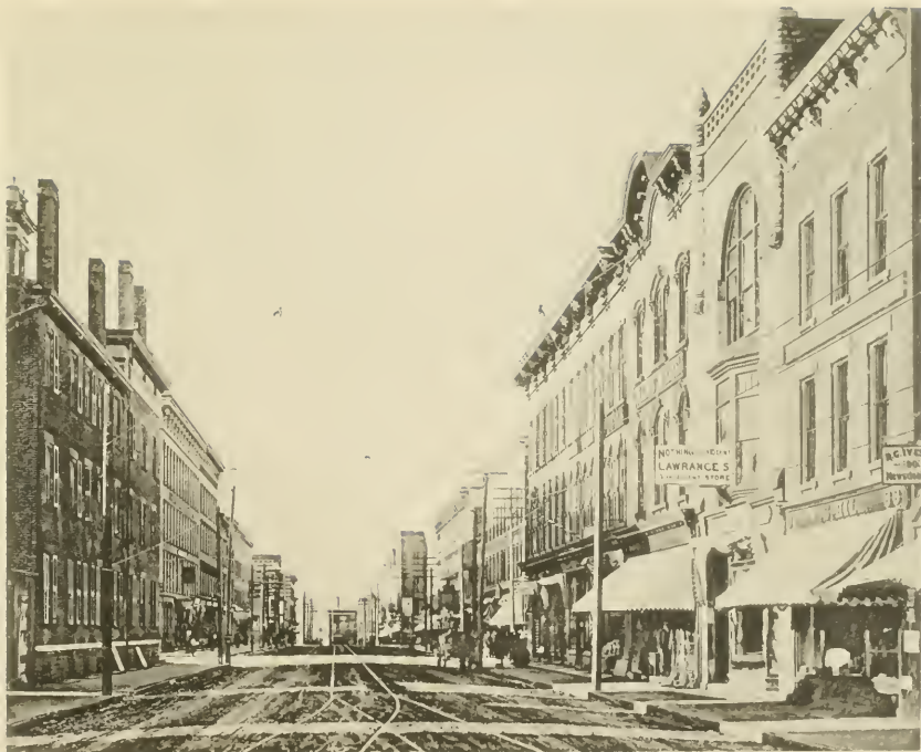
FORD STREET, LOOKING WEST
