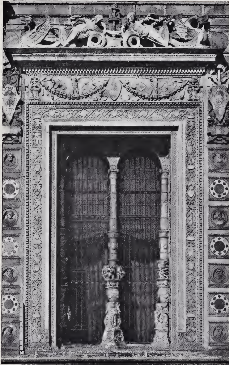
Window in the Façade.
