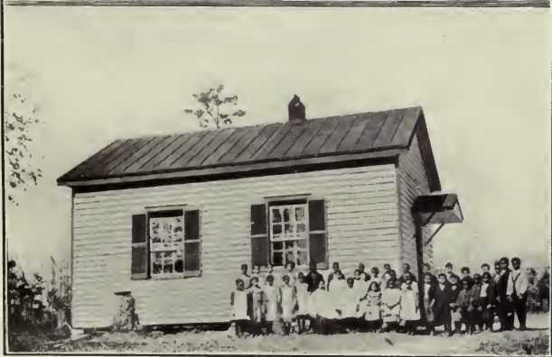
Poplar Lawn School, Va. "Before and After."
