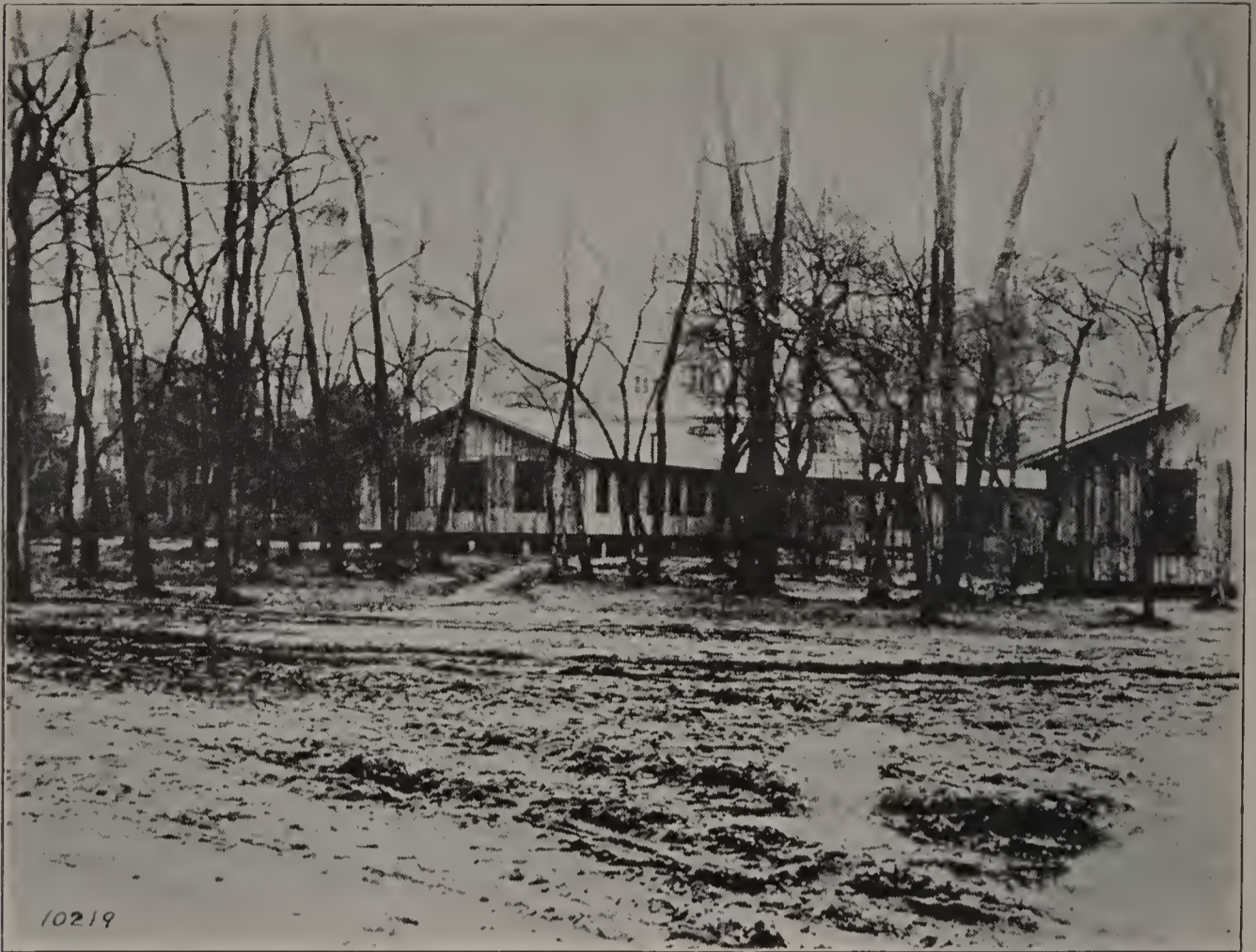
THE LARGE KITCHEN AND MESS HALLS BUILT BY THE 18TH ENGINEERS
