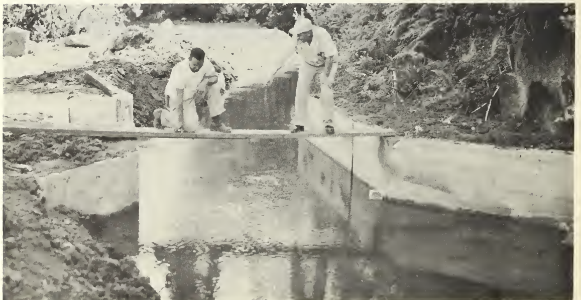
Figure 40.--A concrete structure above the flume on the Lacomb Irrigation District ditch diverts water from Crabtree Creek, subbasin 5, Middle Willamette River Basin, Oreg. SCS photo. 7-938-12
