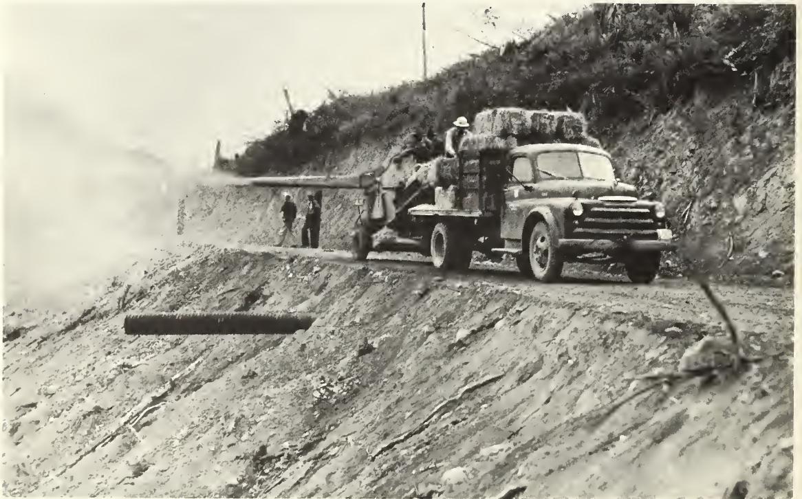
Figure 27.--Straw mulch is being applied to grass-seeded fill slope on this forest road as a temporary soil protective measure. USFS photo.
