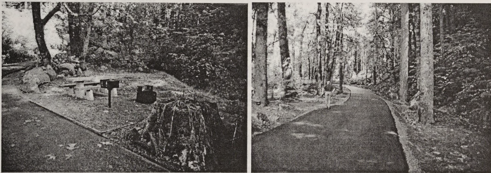
Reconstruction of the East Shore Recreation Site was completed in FY 99
