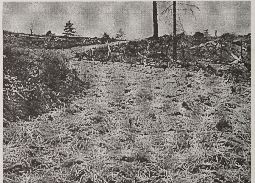
A road decommissioned by ripping, mulching, and seeding
