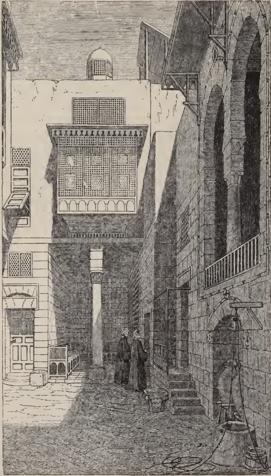
Court of a Private House in Cairo.
