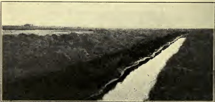
Figure 12.—A Good Drainage Ditch. The first thing to do in reclaiming a marsh is to drain it. This ditch is deep enough to permit drain tile to empty into it. Courtesy of Wis. Agr'l Exp. Sta.
