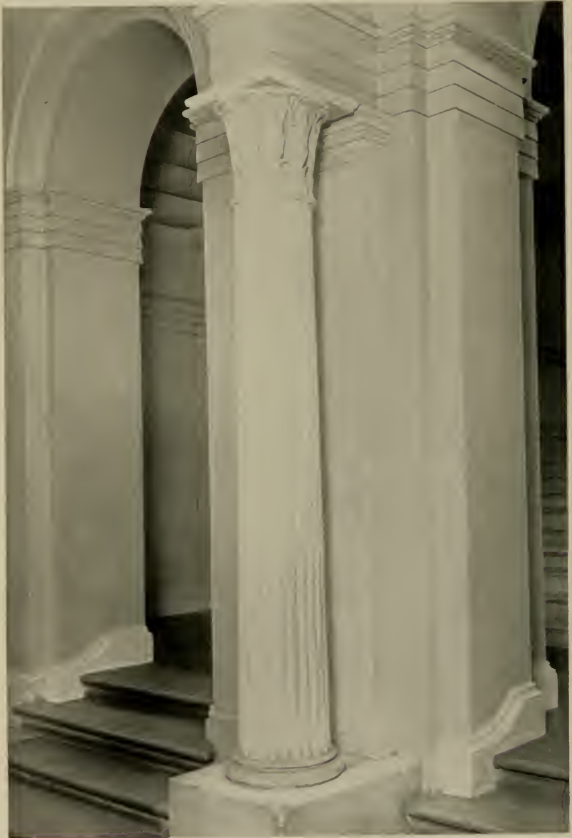
COLUMN IN THE CAPITOL AT WASHINGTON DESIGNED BY LATROBE SHOWING MAIZE MOTIF.
