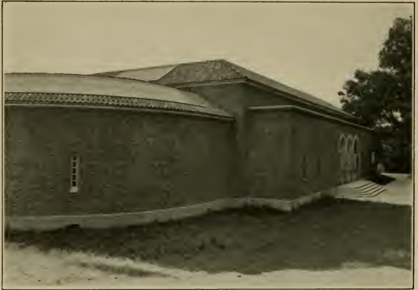
1. SMALL MAMMAL HOUSE AS SEEN FROM THE ROAD.
