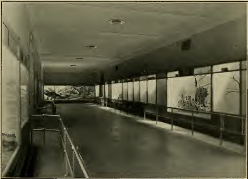
2. INTERIOR OF NEW ADDITION TO BIRD HOUSE.
