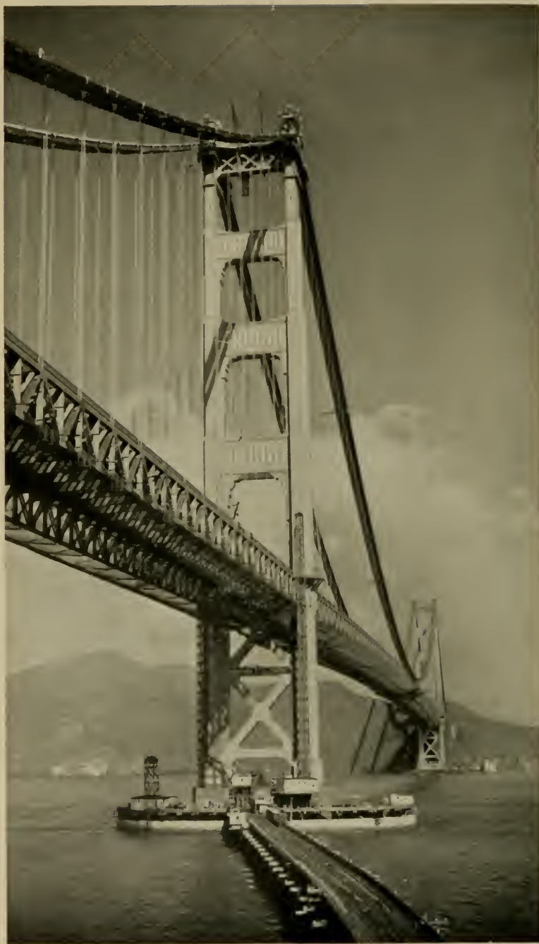
THE SAFETY NET STRETCHED BENEATH THE SUSPENDED STRUCTURE WAS REMOVED AFTER COMPLETION OF ALL WORK.
