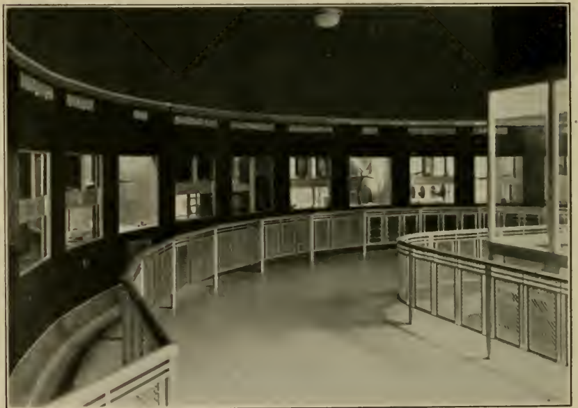
2. INTERIOR OF NOCTURNAL ROOM OF SMALL MAMMAL HOUSE.
