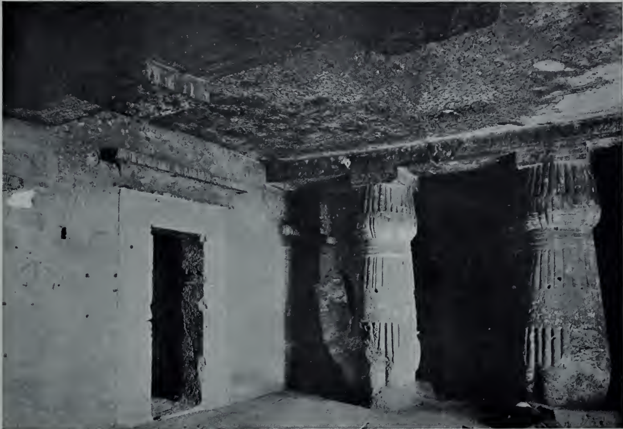
NORTH WALL AND COLUMNS.
