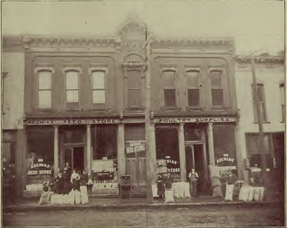
Front View of Our Seed Stores, 106-108 E. Main St., which have over 11,200 Square Feet Floor Space.
