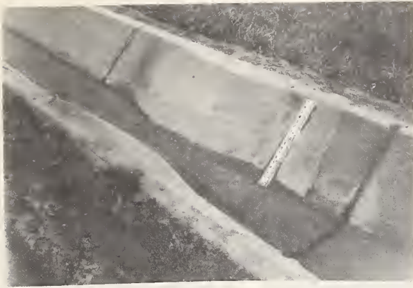
Figure 6. Cast trapezoidal flume using the ditch invert as the flume bottom.
