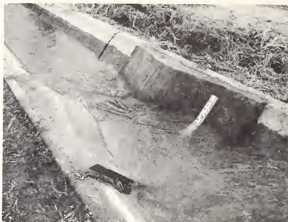
Figure 8. The flume shown in figure 7 with a flow of 1.2 cfs, operating at a submergence of about 70%.
