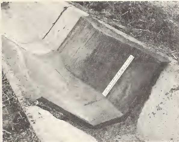
Figure 7. Trapezoidal measuring flumes with a raised bottom cast in a concrete ditch.
