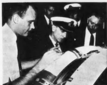
ACTIVITY AT CAPE KENNEDY—Top panel, left to right: Engineers J. B. Wynn and R. W. Kenyon examine a reradiating antenna which permits a missile-carried transponder to be checked out while missile is in launch tube; D. J. Leffler uses telemetry data to assess flight test results; E. M. Hlavaty and
