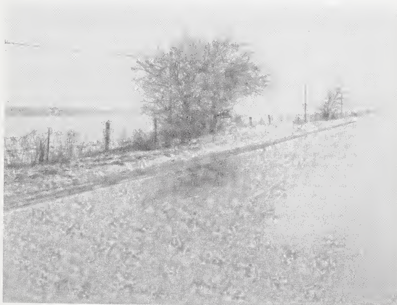
Flooding Along State Route 714 February 3, 1982
