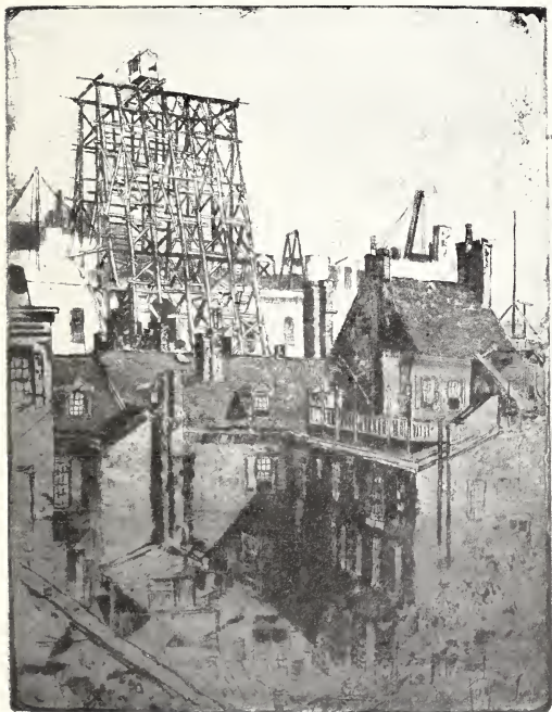
Last of the Scaffolding. (Philadelphia Public Buildings.)
