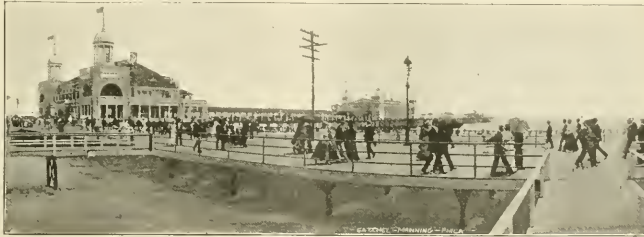
STEEL PIER FROM BOARDWALK.
