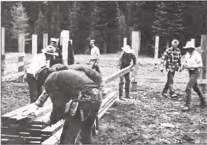
Volunteers hard at work building corral.
