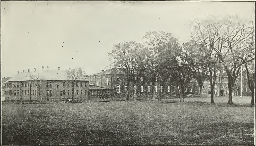
CONNECTICUT STATE PRISON—Situated at Wethersfield.
