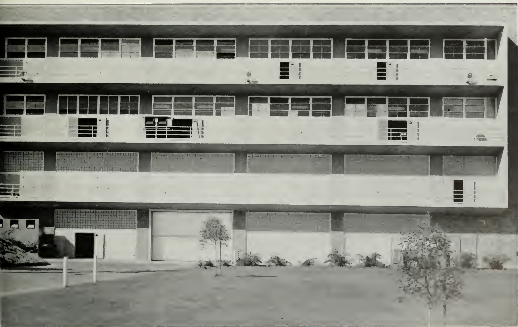
The recently completed Engineering Building has been an important addition to the growth of the department.
