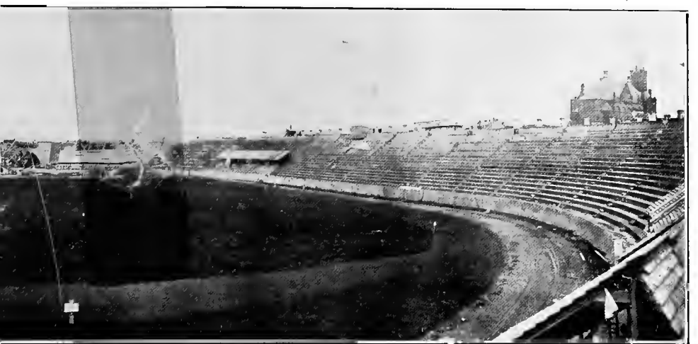
the picture at the furthest extremity. An idea of the magnitude of the structure may be
