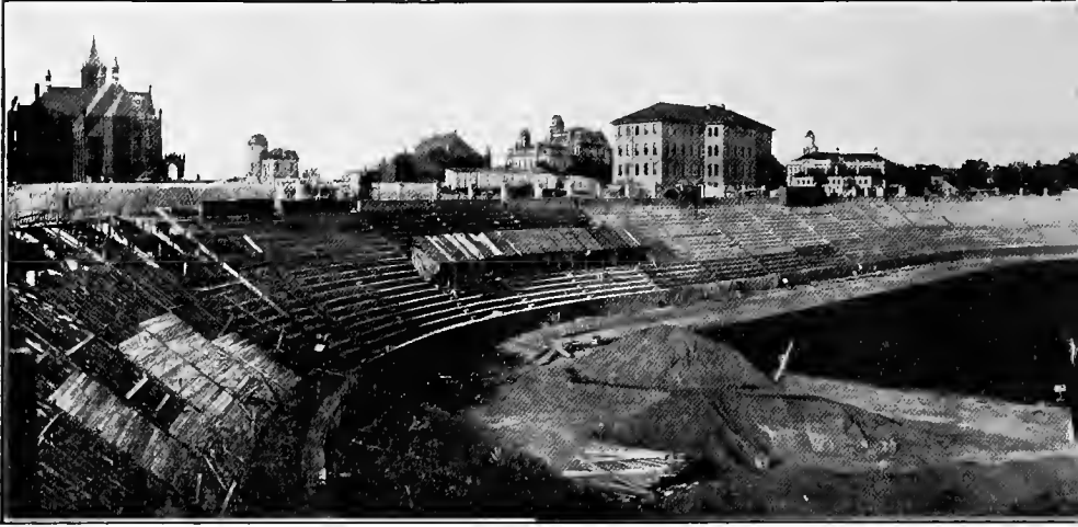
View looking East showing the Gymnasium Tunnel
