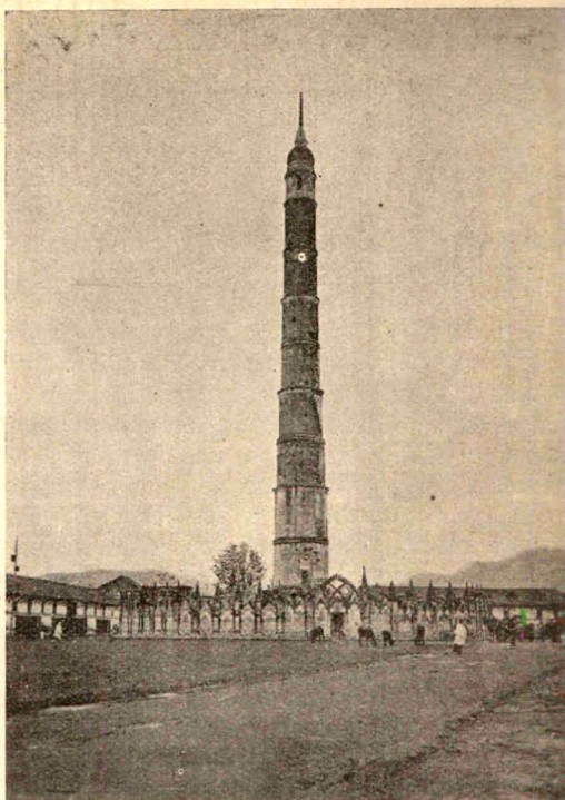
Dharara or Tower of Bhimsen Erected by General Bhimsen Thapa
