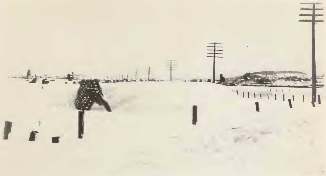
FIGURE 1. END VIEW OF SNOW FENCE WITH RESULTANT DRIFT, THE PROTECTED ROADWAY IS AT THE RIGHT BEYOND THE TELEGRAPH POLES.
