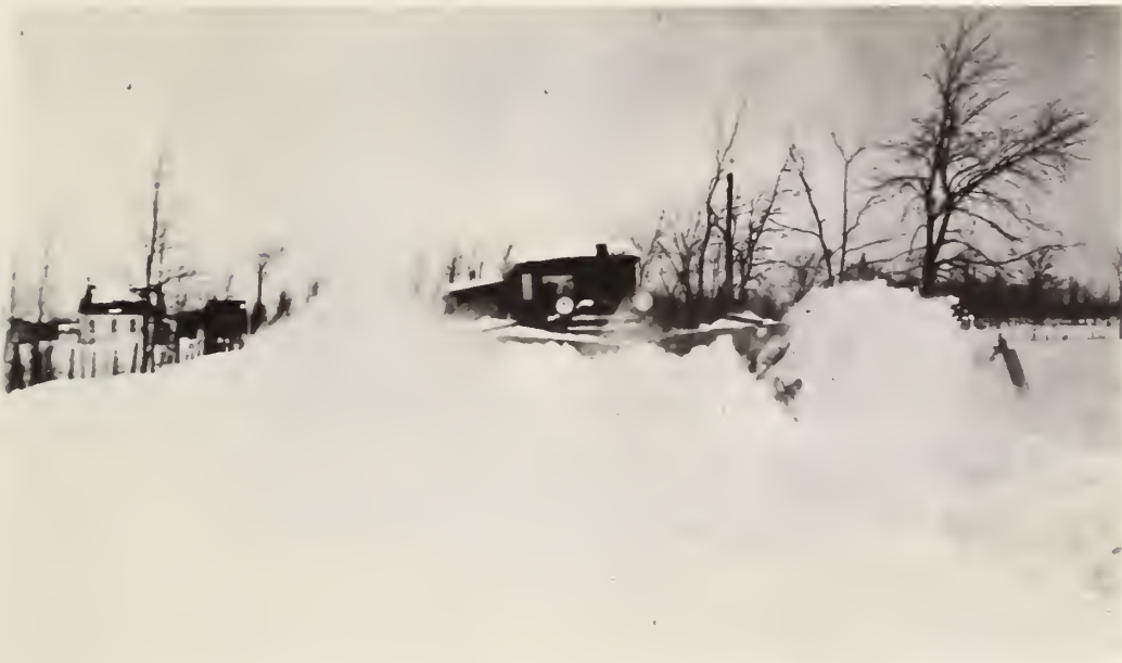
FIGURE 8. A ROTARY PLOW OPENING A PASS THROUGH THE SECTION OF ROAD SHOWN IN FIGURE 7.
