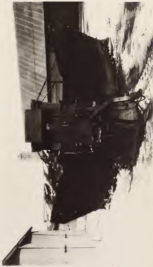
FIGURE 3. A DISPLACEMENT PLOW FOR TRUCK MOUNT. ONE OF MANY DESIGNS SUITABLE FOR TRUCK MOUNT.
