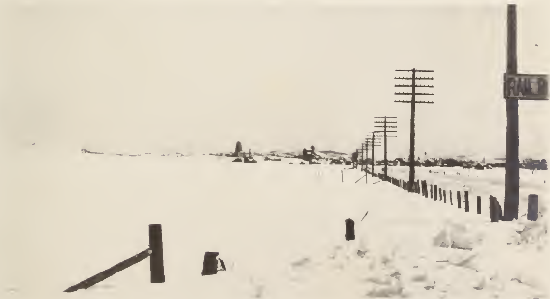
FIGURE 2. VIEW OF THE LEE SIDE OF DRIFT SHOWN BY FIGURE 1, WITH THE ROADWAY COMPARATIVELY FREE OF SNOW.
