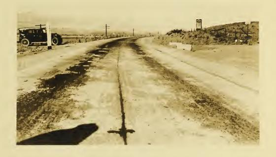
FI WE 1-(T.P)- Typical Scaling on a concrete pave of the Luinvis, surface treated with calcium chloride.
