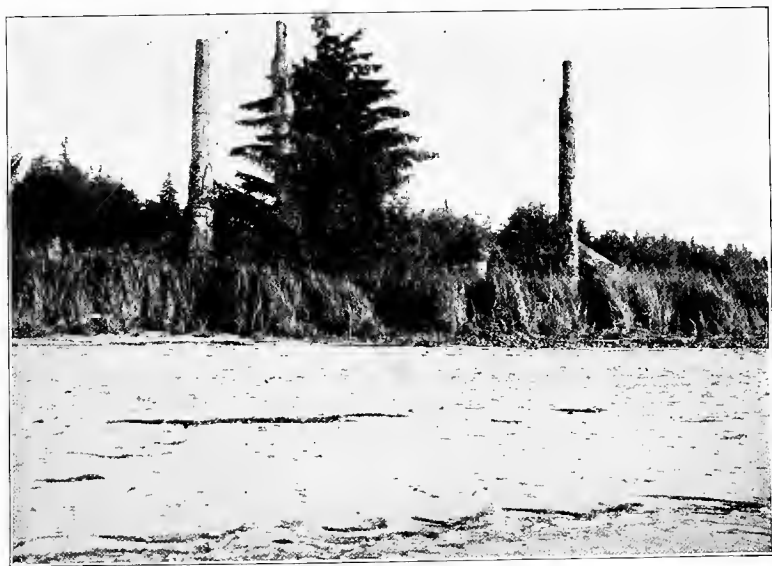
Ruins of old Communal House at Kung. October 31.
