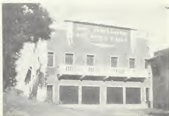
A cooperative plant of the CÔTES D'AGLY Wines (Pyrénées Orientales). There are about 1,000 wine cooperatives in France.
