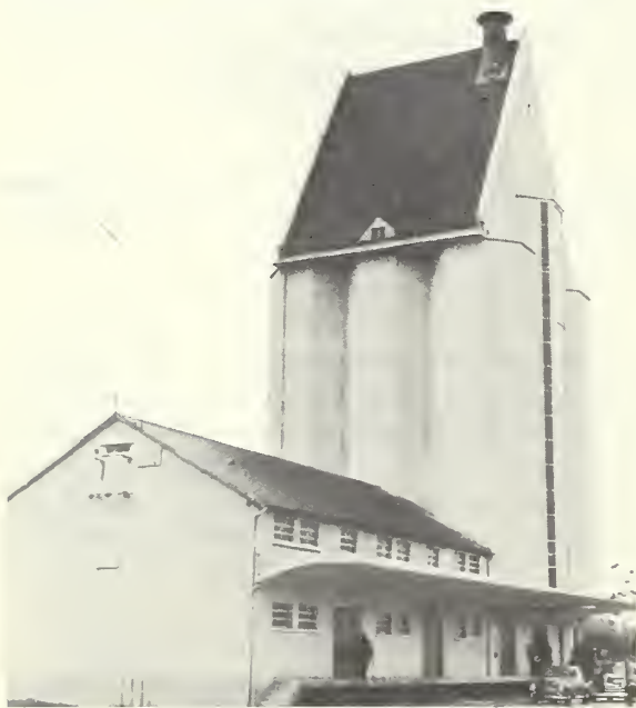
A 3,800-ton grain elevator at SAINVILLE, in the rich Beauce area, southwest of Paris. About 70 percent of the grain storage in France is operated by co-ops.
