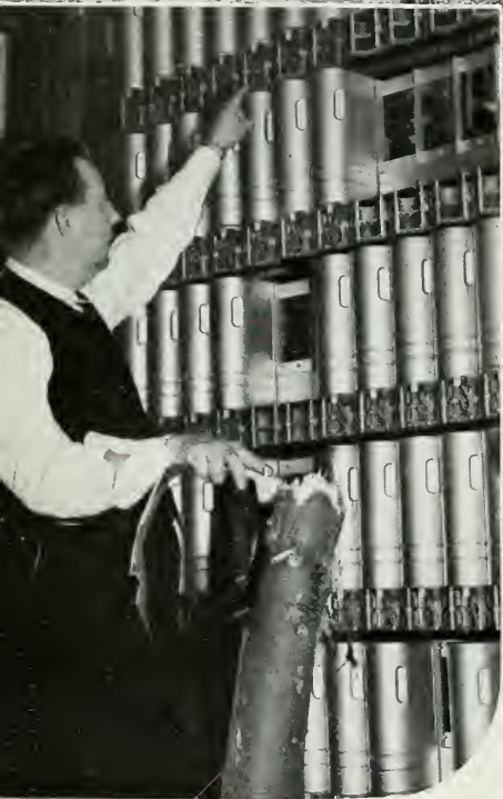
A 3-foot section of tree trunk plummeted through the roof of the Deep River, Conn., central office and bounced up to the top row of dial equipment.
