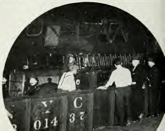
An aerial cable truck being secured in a gondola for the ride to the devastated area.
