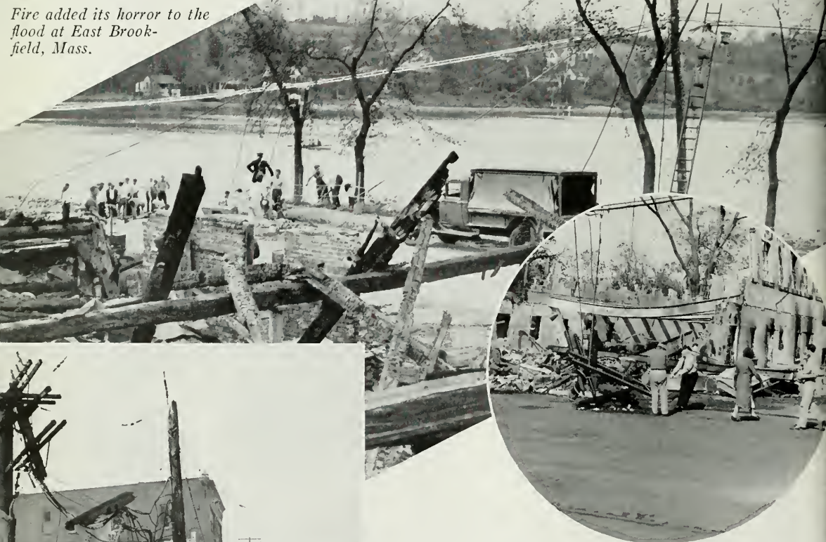
Flames melted telephone cables, adding to the general destruction of plant, as here at New London, Conn.
