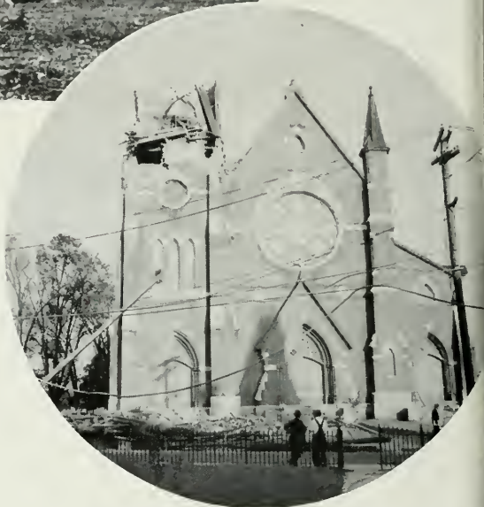
The steeple of this Willimantic, Conn., church crashed through a local telephone cable.
