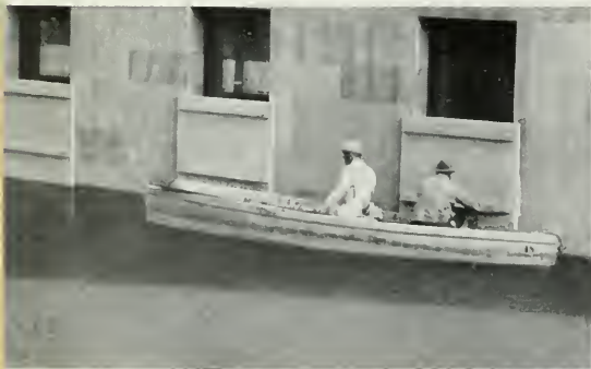
After the great flood of 1936 in Hartford, Conn., bulkheads were built for all doors and windows of the telephone building nearest the river. The picture at the right shows how they kept the water out last month; the small picture above shows boatmen patrolling the outside of the building, with water several feet above the first floor windowsills.
