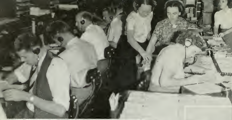
Below: Patching cords at the New England section of the Long Lines telegraph testboard in New York City immediately after floods and hurricane made necessary the rerouting of circuits
