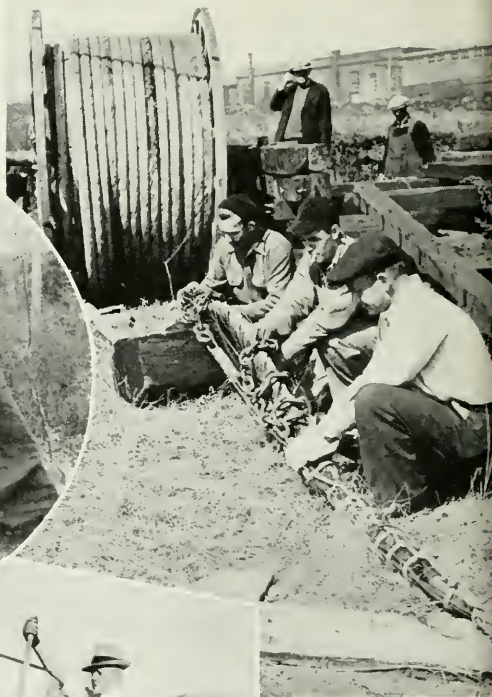
Right: A new submarine cable to replace one under the Taunton River in Massachusetts which was severed by a dragging anchor. Circle: Control station near Keene, N. H., for the short wave radio circuits which temporarily bridged the gap to Boston.
