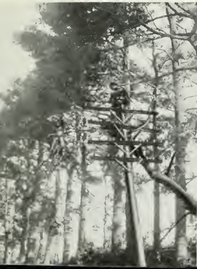
Splicing temporary twisted pair into an important open wire toll route east of New London, Conn.
