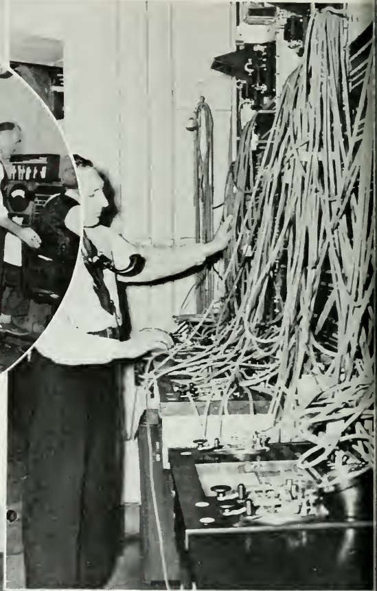
Below: Patching cords at the New England section of the Long Lines telegraph testboard in New York City immediately after floods and hurricane made necessary the rerouting of circuits
