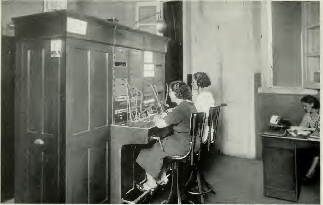
BELL SYSTEM OVERSEAS SERVICE REACHES PLACES SMALL AS WELL AS LARGE. THIS SWITCHBOARD IN CIUDAD TRUJILLO, DOMINICAN REPUBLIC, CONNECTS WITH THE A. T. & T. STATION AT MIAMI, FLA.
