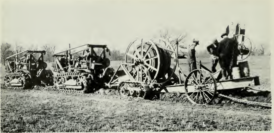
FIG. 2. PLOWING IN BURIED CABLE ARMORED AGAINST NATURAL AND MAN-MADE HAZARDS.
