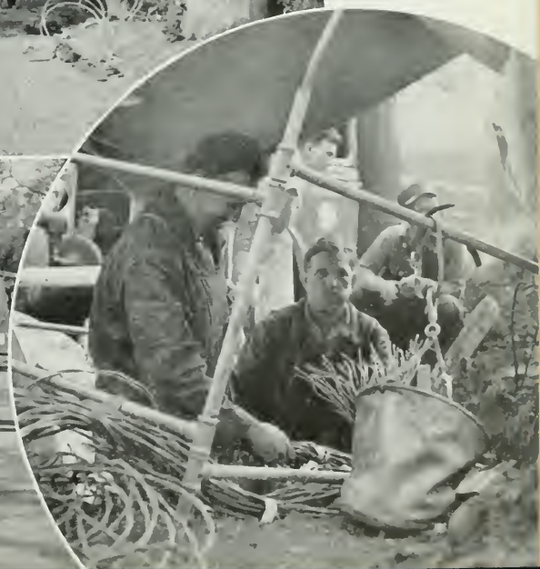
Below: Splicers at work at the Atwoodville Long Lines cable break.
