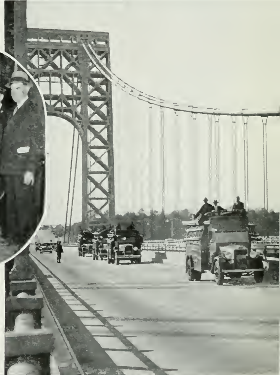
The first contingent of New Jersey Bell construction crews crossing the George Washington Bridge on their way to help their fellow workers in the east.
