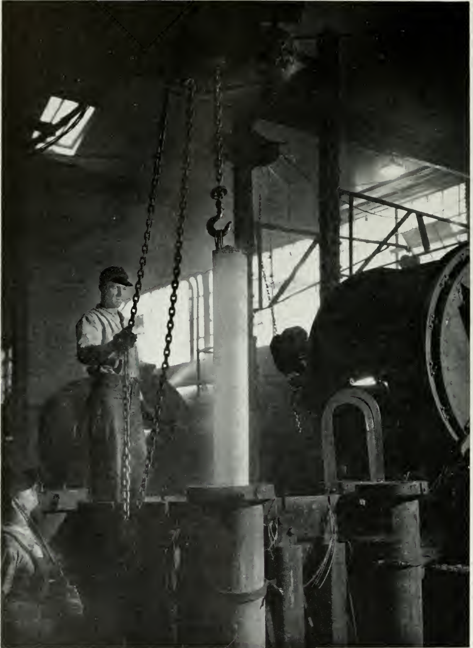
This gleaming, molten billet is lifted red hot from its mould by the electric chain hoist. This is one of the processes in reclaiming used metals and returning them to the telephone plant again, in this particular case as bronze drop wire which will be made from the billet.
