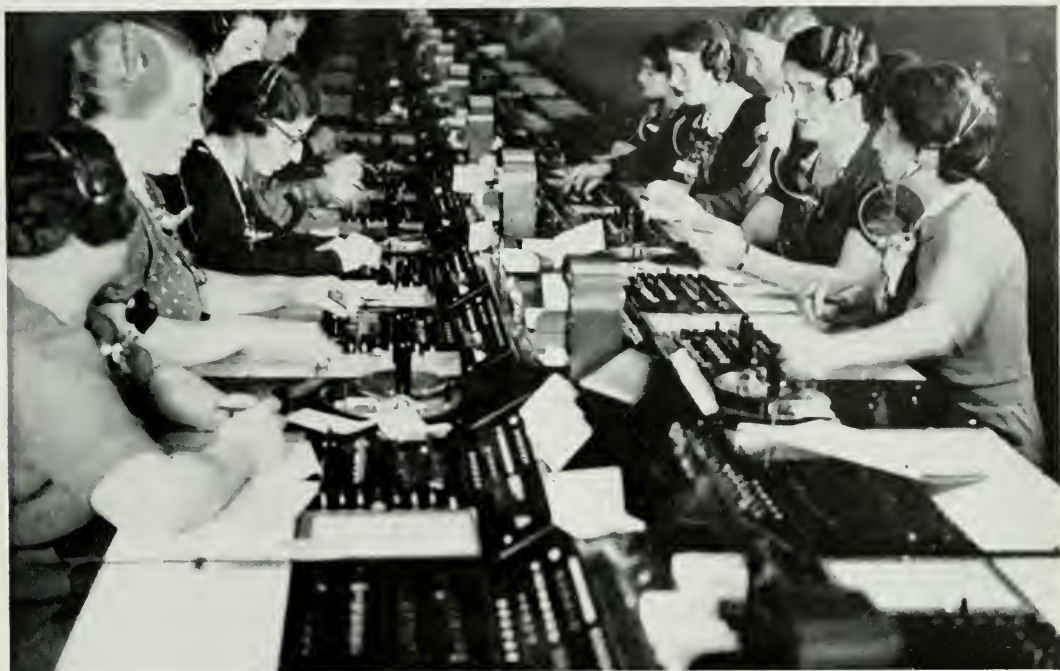
A SECTION OF THE LONG DISTANCE SWITCHBOARD AT AMSTERDAM, THE NETHERLANDS.
