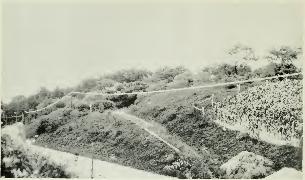
FIG. 7. PART OF THE MECHANICSBURG-SHEPHERDSTOWN, PA., TOLL CABLE, WITH THREE-HUNDRED-FOOT SPANS. SHOWING HOW IT IS POSSIBLE TO UTILIZE HIGH SPOTS IN THE CABLE ROUTE FOR PLACING SHORT POLES.
