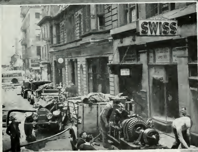
The fire engine at the left is pumping out man-holes in Providence, R. I., while the generator in the foreground is providing emergency power for the New England Company's central office.
