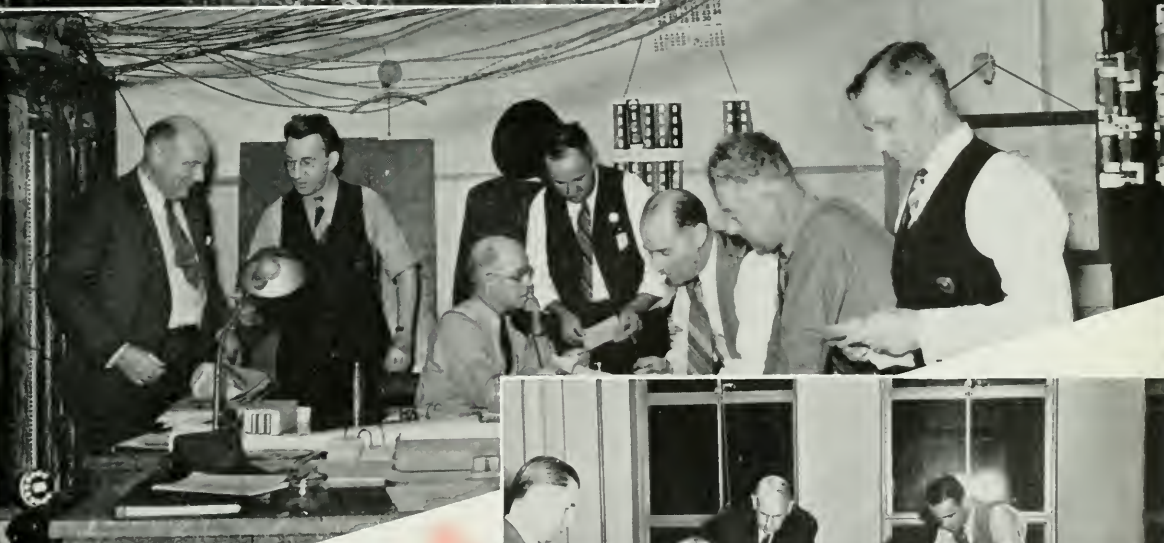
Headquarters of the Installation Department in Providence, R. I., directing restoration of service under difficult conditions.
