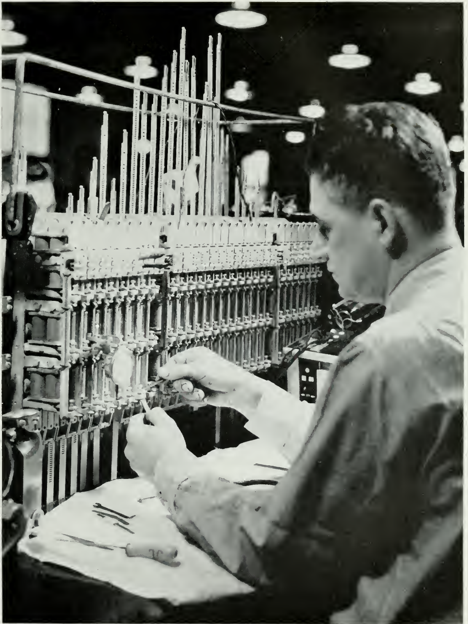
Adjusting clutches on friction roll drives on panel dial exchange equipment. These drives move the selector rods which make the desired connections.
