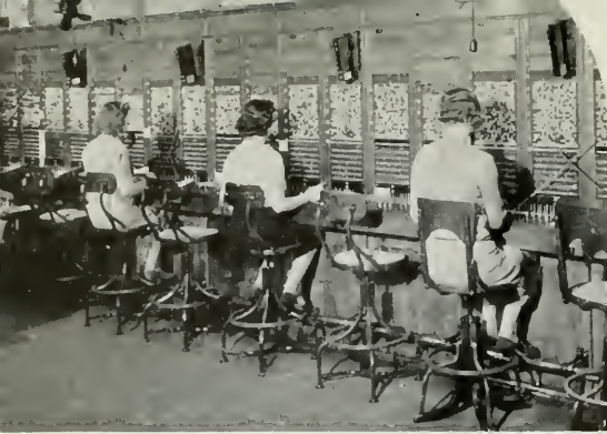
Each white plug at this switchboard at Keene, N. H., shows a line out of service. After the hurricane, only 50 out of 1853 lines were working.
