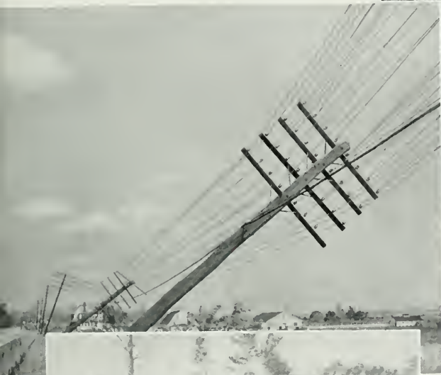
Where there were no trees, pole lines sometimes survived intact the fury of the wind, as in the case of this line at Rutherford, N. J.
