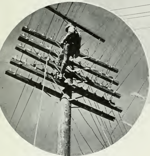
Splicing temporary twisted pair into an important open wire toll route east of New London, Conn.
