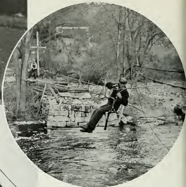
A Long Lines lineman rides temporary strand where the Mount Hope River took out important New York-Boston cables.
