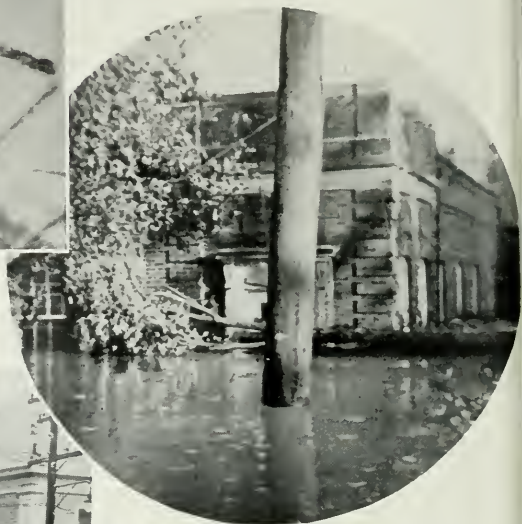
This view toward the front door of the central office at Orange, Mass., shows why the operators had to quit their positions.
