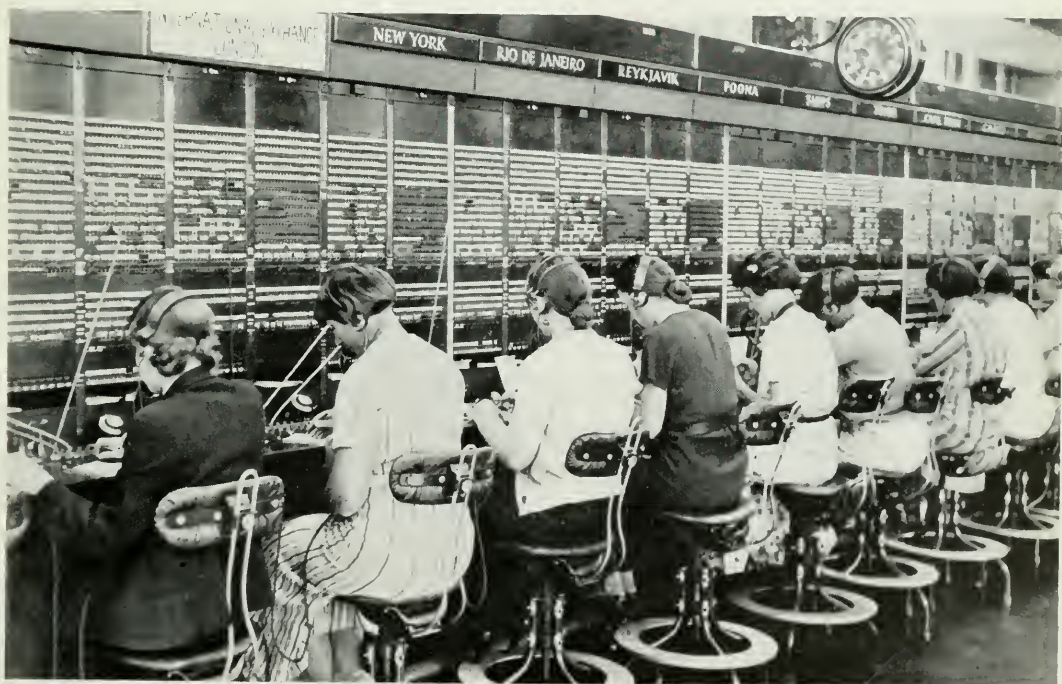
THE INTERNATIONAL SWITCHBOARD IN LONDON, WHERE OVERSEAS RADIO TELEPHONE CIRCUITS ARE LINKED TO THE WIRE LINES TO OTHER PARTS OF GREAT BRITAIN AND TO THE CONTINENT.
