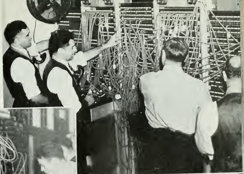
Below: These patches at a Connecticut long distance telephone testboard show how messages were routed through on circuits still working.
