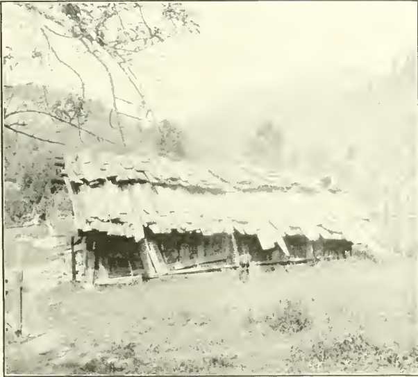
KAROK HOUSE, SIDE VIEW, SHOWING DOUBLE PITCH AND RAGGED SHINGLING OF ROOF
