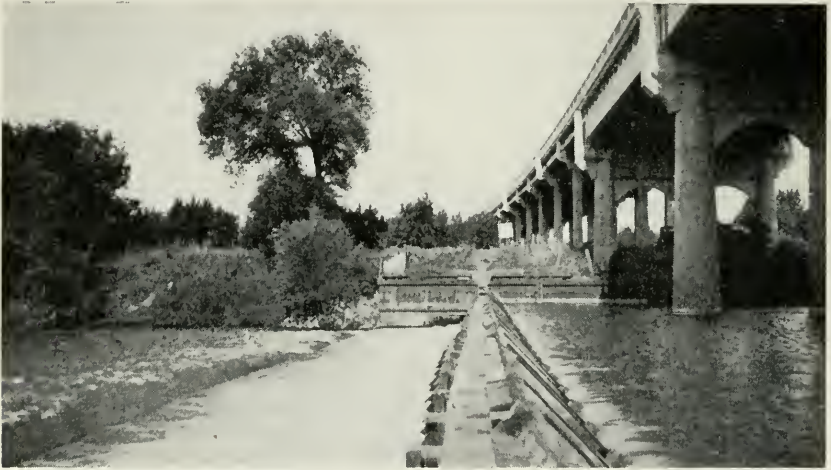
FIG. 37. The Modesto Weir on the Tuolumne River. The fishway is in the center background. Photograph by Paul R. Needham.
