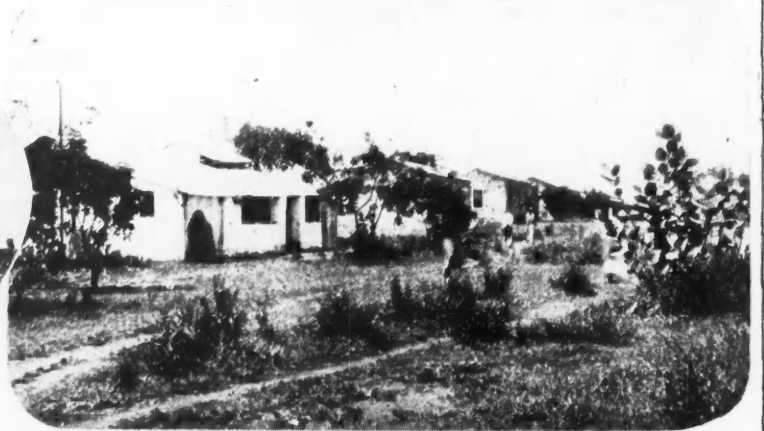
Assay office and houses built by the German company which worked the mines at Sekenke, 1909-1915
