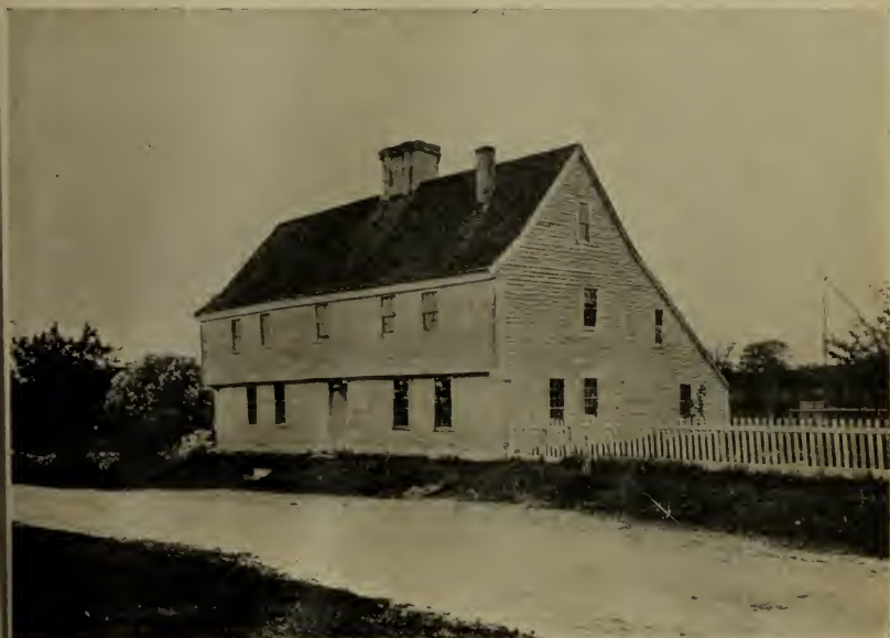
BENNETT-BOARDMAN HOUSE, OAKLANDVALE
