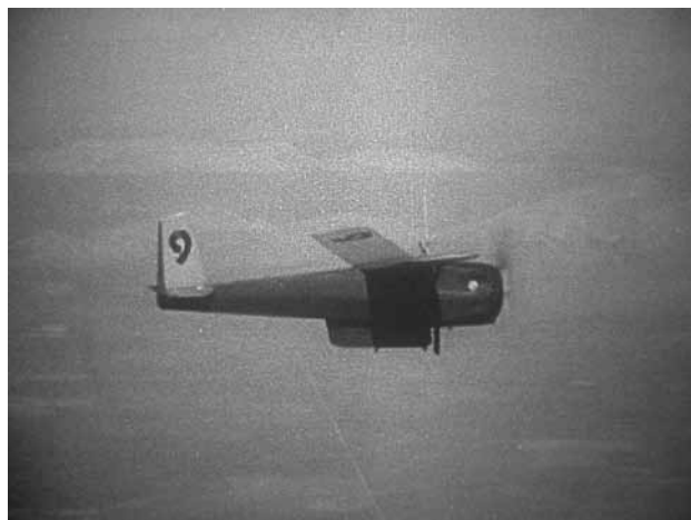
The General Motors A-1 flying bomb was a conventional high-wing monoplane powered by a 200-hp piston engine. It was launched from a four-wheeled dolly, and could carry a 500-lb bomb over a distance of 400 miles. Initial tests between 1941 and 1943 were not very successful because basic problems of inadequate control had not been resolved. AFFTC History Office
